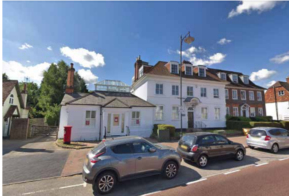
Photo 2 - View of the front elevation from High Street
