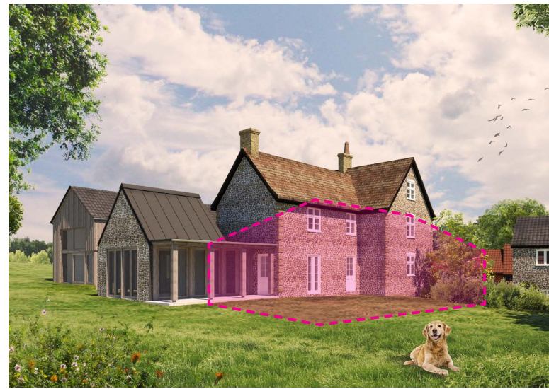
Fig 1. Proposed view from the south west looking at the listed farmhouse. Outline of the removed conservatory is shown to indicate the extent it inhibits the view of the farmhouse.
