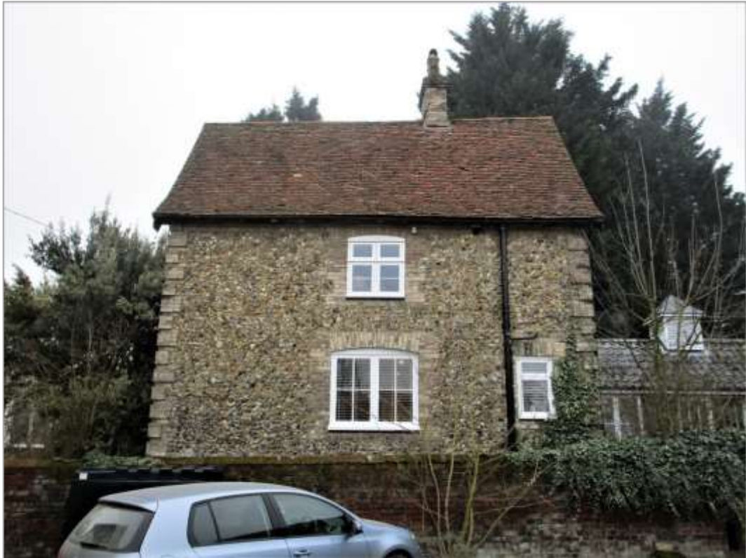
Fig. 12: The listed farmhouse does not have a 'front' elevation in the sense of an entrance elevation. The current entrance is via the c.1990 link (just visible to the right). The early OS maps suggest a path approach to a door on the S side, in an area now rebuilt. This photograph shows the E elevation, facing towards the farmyard. It has two central windows and a small modern off-the-peg window to the right. The chimney stack is placed off-centre and is of C19 date.
