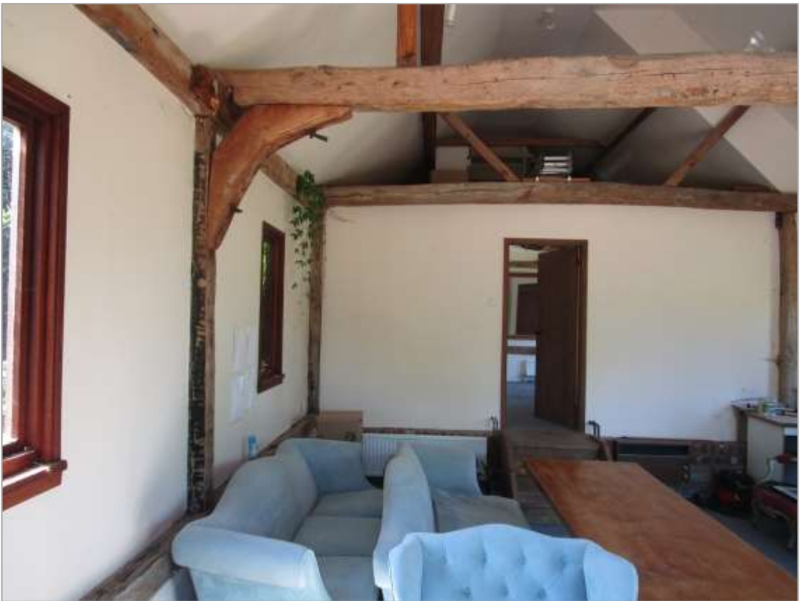
Fig.28: Interior of Building D
