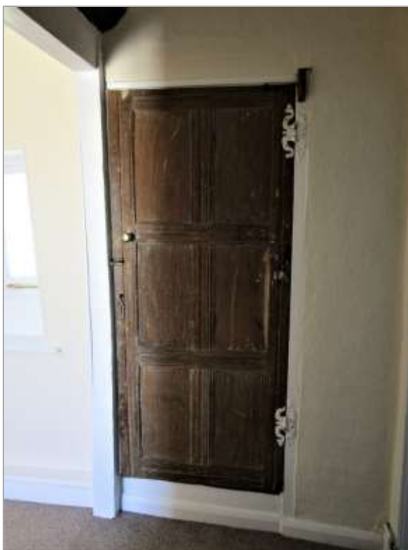
Fig. 18: C17 door with elaborate hinges, cross wing first floor, by stair to second floor
