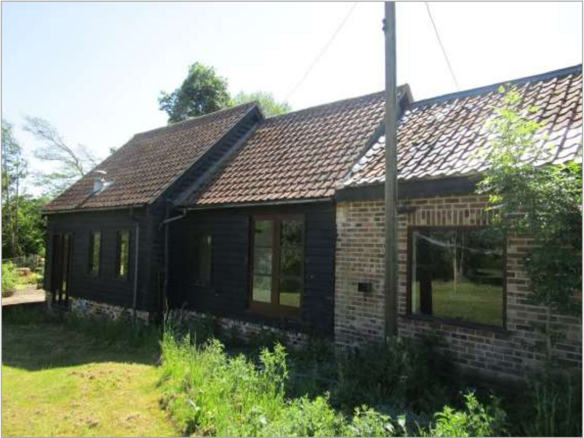
Fig. 27: Building D from NE
