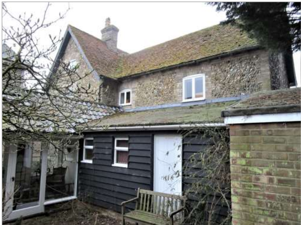
Fig. 15: Behind the link, a black weatherboarded lean-to structure is of C20 date. Alongside, a modern brick structure with shallow lean-to roof is in the small courtyard garden.
