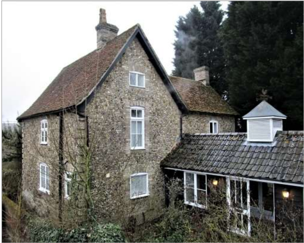
Fig. 14: The N and E elevations viewed from the upper floor of the N range, with c1990 link to right. The listed building displays a variety of window types (consent was given for the replacement of most of these in 2016).
