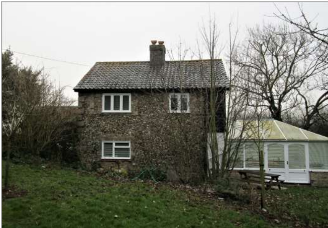
Fig. 25: The W elevation of the cottage has mid-C19 flint walling and brick quoins. The window openings are modern. The building has been rebuilt and enlarged to the S (see painted brick and weatherboarded section beyond the brick quoins to right).
