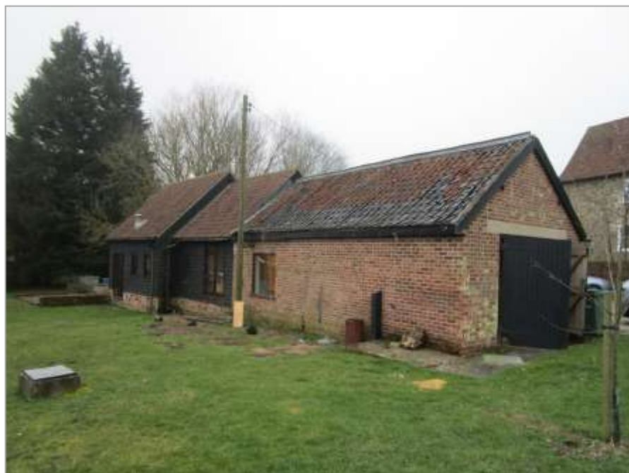
Fig.30: Building E from NW.
