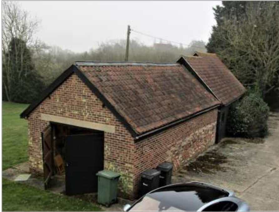
Fig. 29: Building E viewed from upper floor of N range. It incorporates part of an older brick wall at the bottom, but is otherwise modern.
