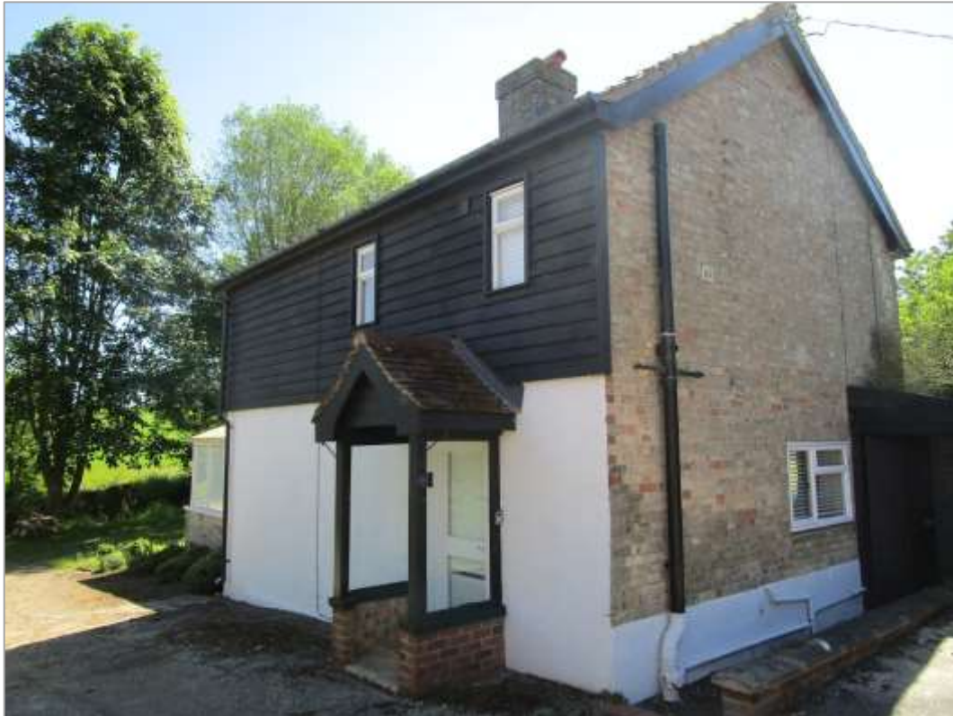
Fig.24: The cottage seen from the farm courtyard to N
