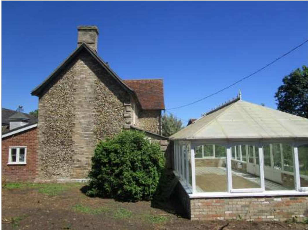
Fig. 16: The modern conservatory extends well beyond the line of the rear range. The W gable end of the rear range is of brick and flint, blind except for one modern ground floor window. On the SW corner the brick quoins are proud, reflecting the subsidiary nature of the N elevation of this range. To the left is the Fletton brick return of the C20 weatherboarded lean-to addition.
