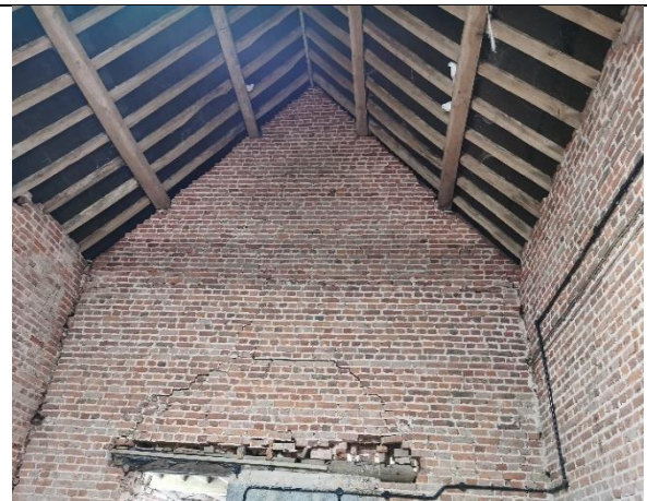
S1 – Internal of central section looking SW.
