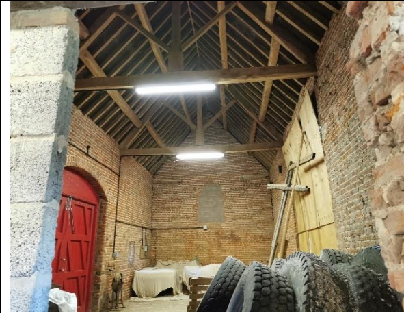
S1 - Internal of central section looking NE.
