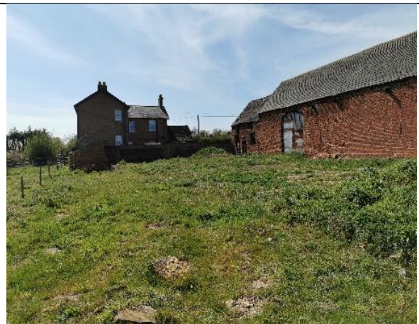
Habitats – Old courtyard area with fragmented walls adjacent to S1.
