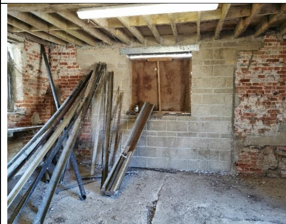
S1 – Internal SW ground floor.
