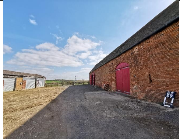
S1 - Northern aspect looking east.
