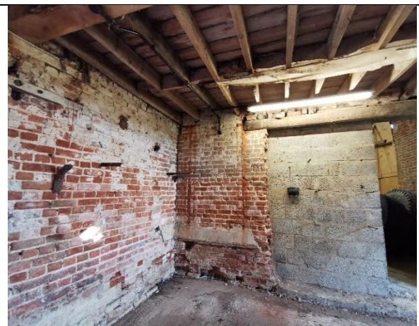
S1 – Internal SW end of looking NE.
