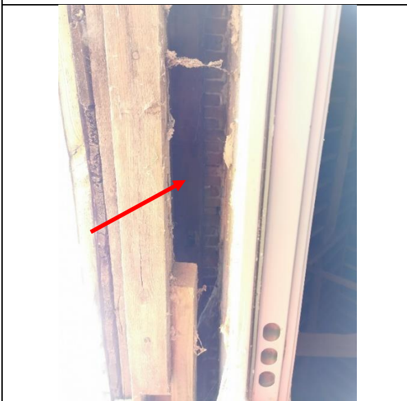
TN33 Cavities behind metal roller shutter door S2.
