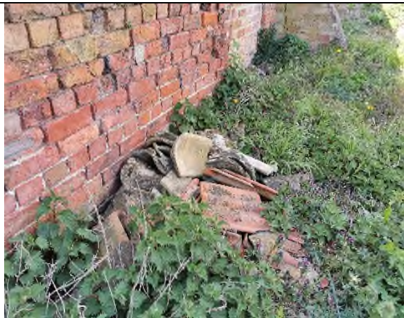
Piled roof tiles - TN4.
