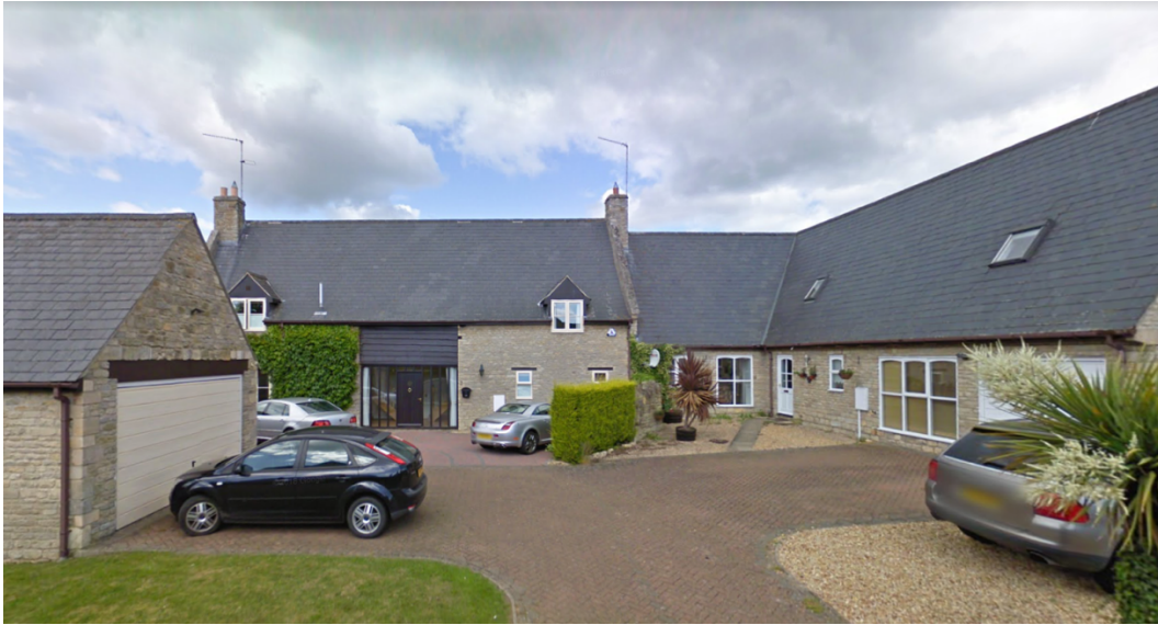
Fig 1. Front elevation of Hayloft 2 and 3 as seen from the road.
