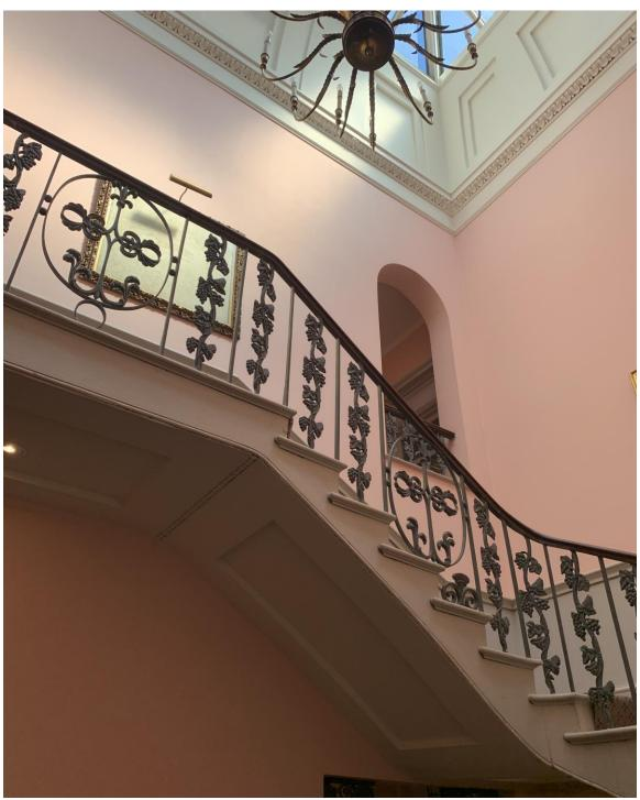
This shows the quality and design of the main staircase rising through the centre of the building, shallow treads, highly decorative balusters, lit by a timber roof lantern.
