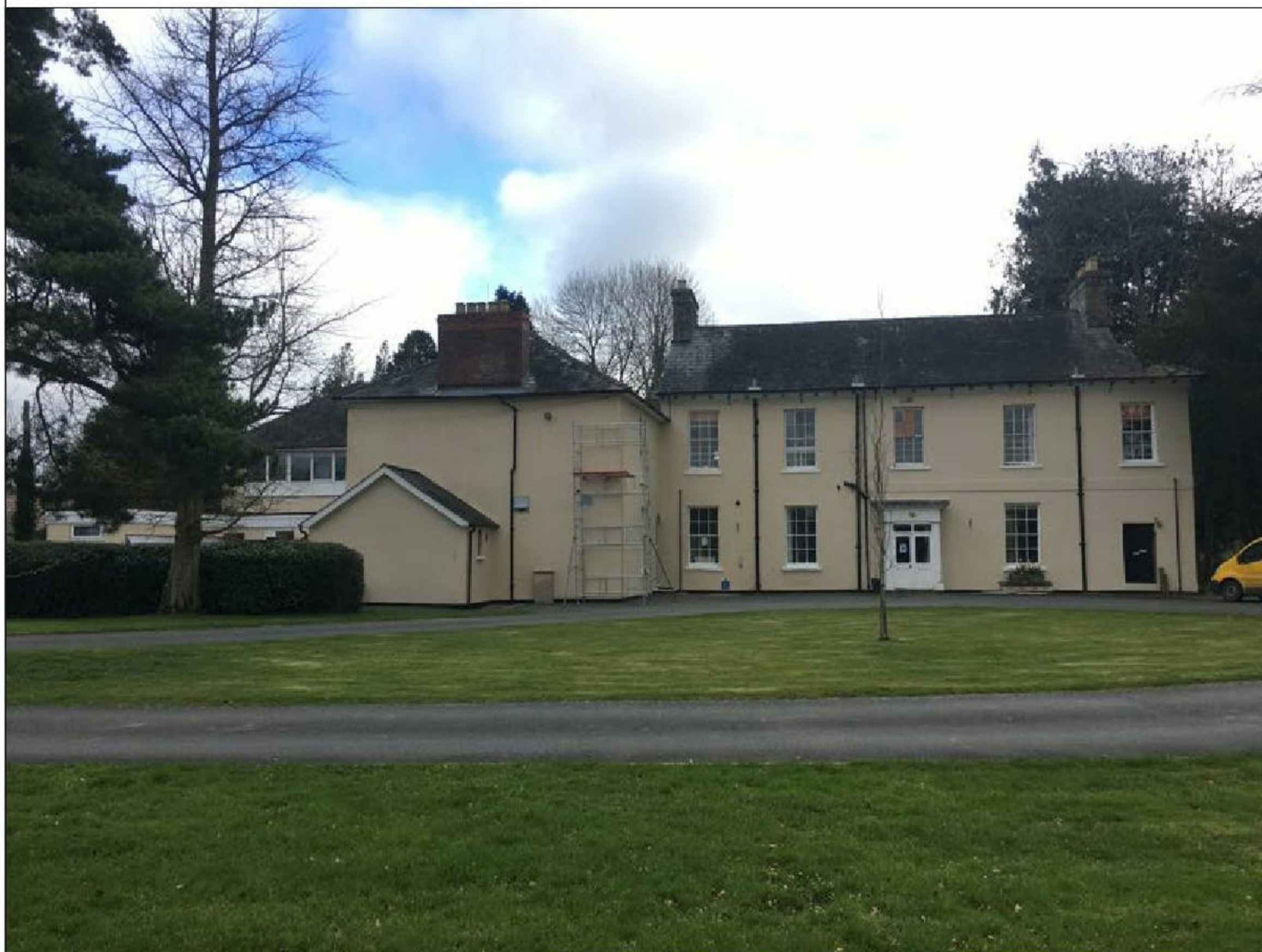
Photo Location - West Elevation image a
