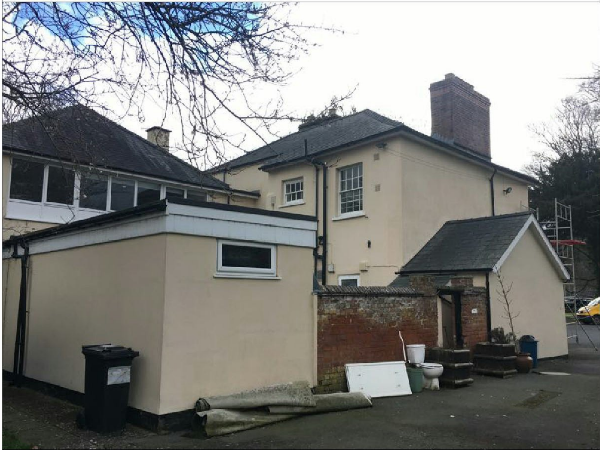
Photo Location - West Elevation image f
