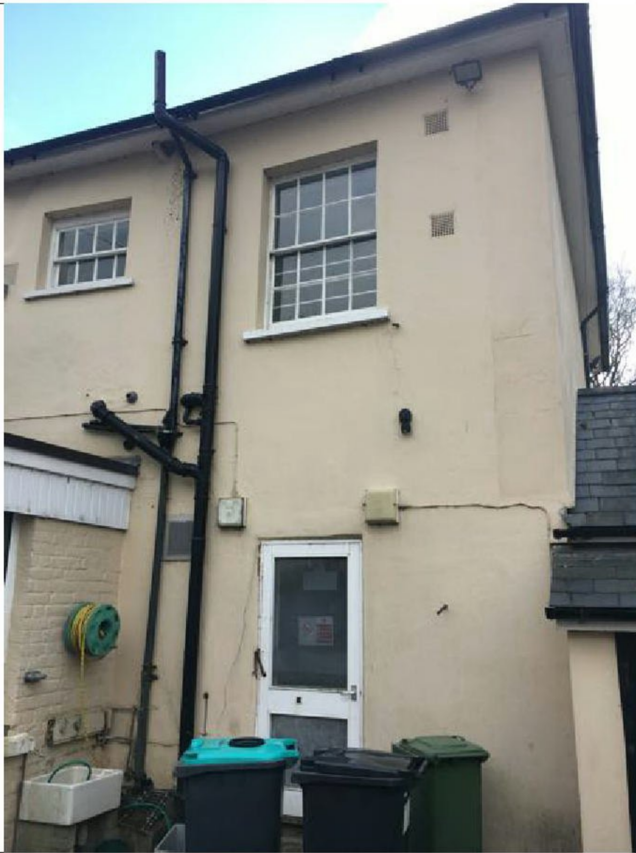
Photo Location - West Courtyard c
