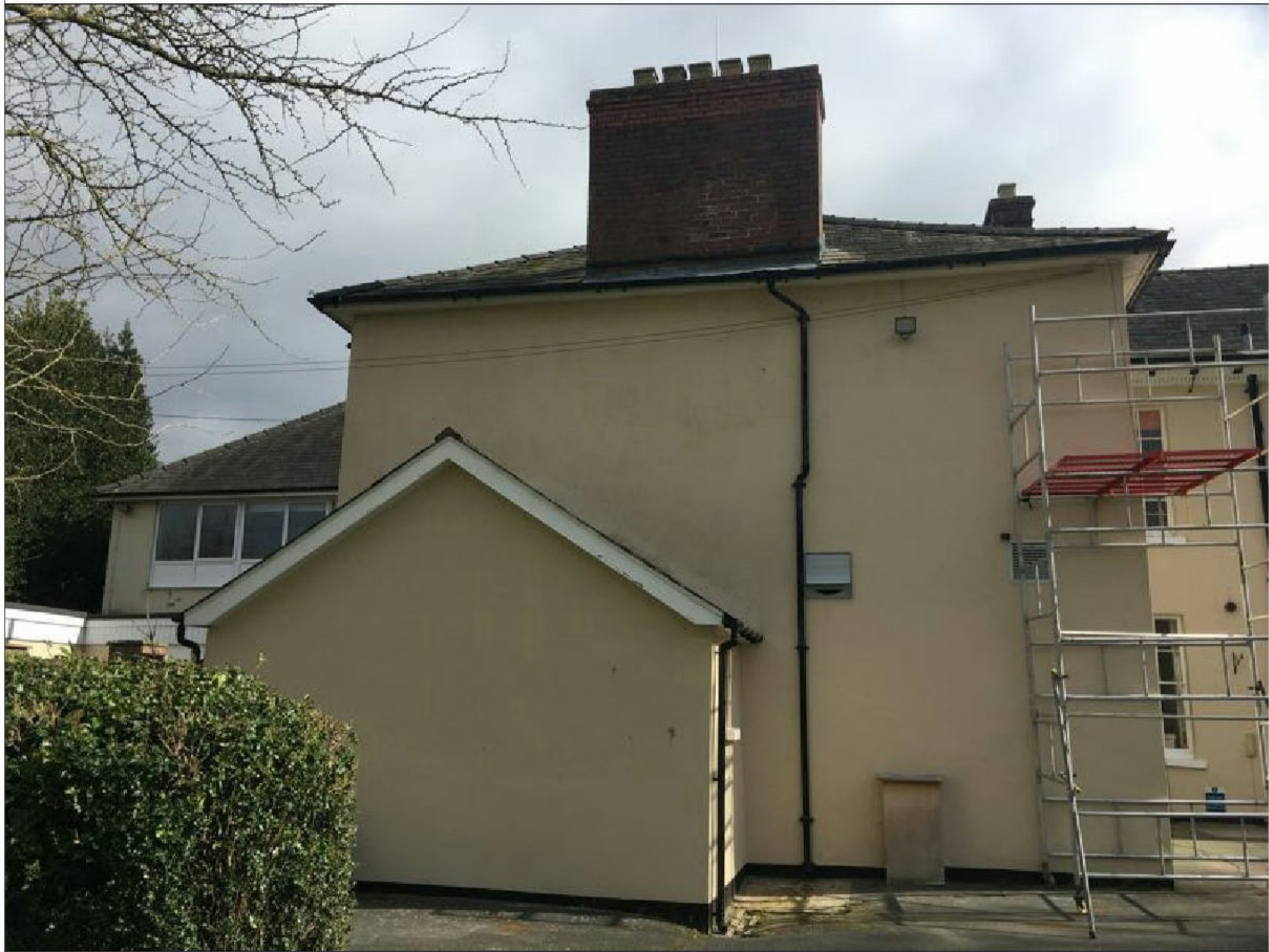
Photo Location - West Elevation image c
