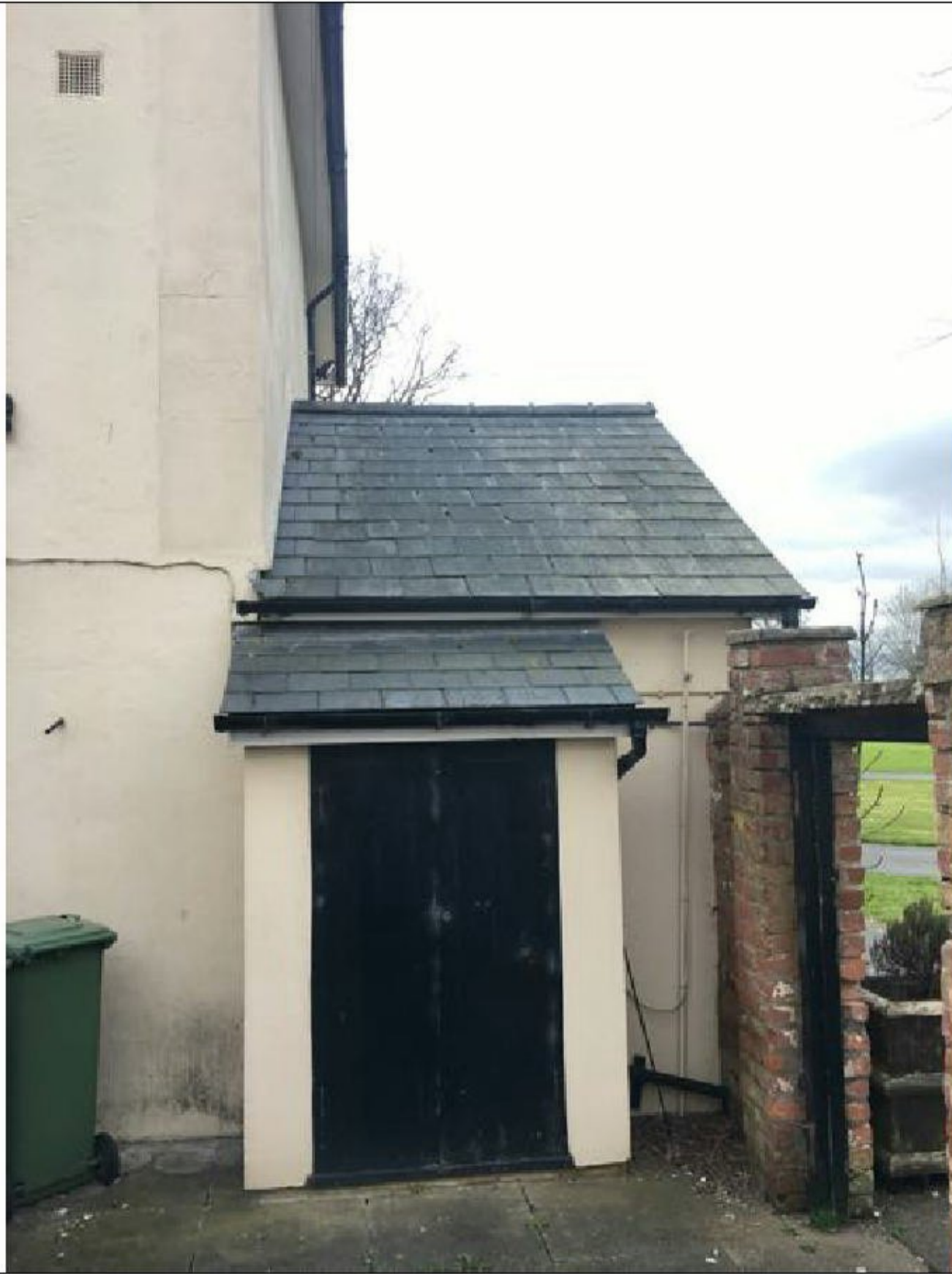
Photo Location - West Courtyard d
