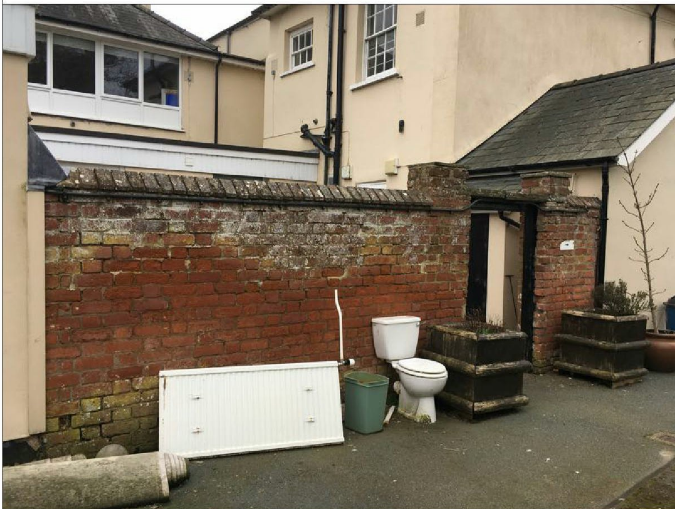
Photo Location - West Courtyard e
