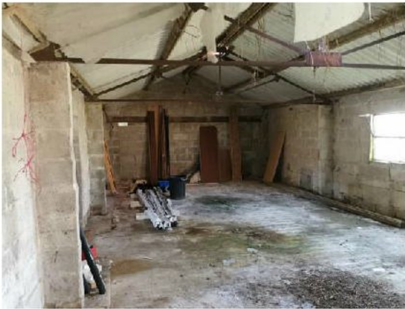
Photo 7. Showing the interior of building 3
