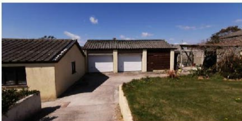
Photo 1. Showing the northern end of the buildings and garage
