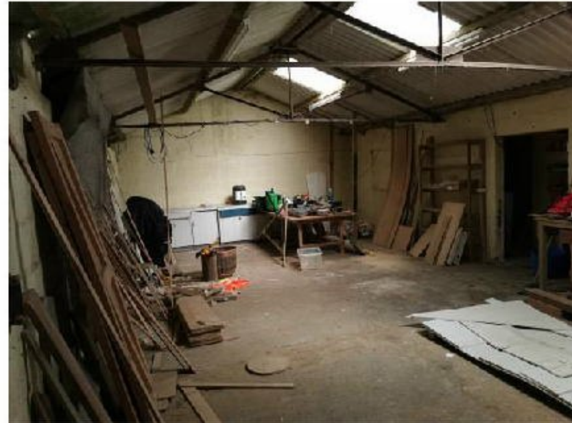
Photo 8. Showing the interior of building 4
