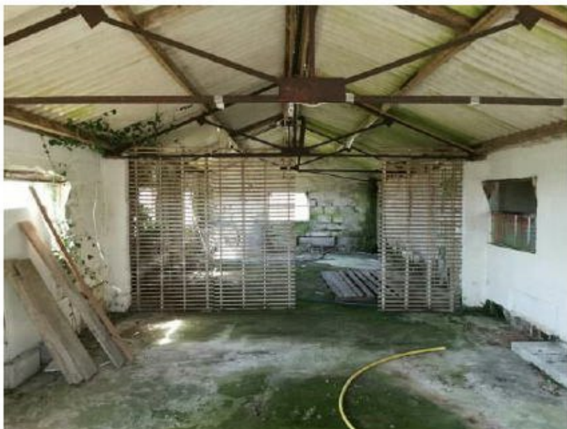
Photo 5. Showing the interior of the southernmost building (1)
