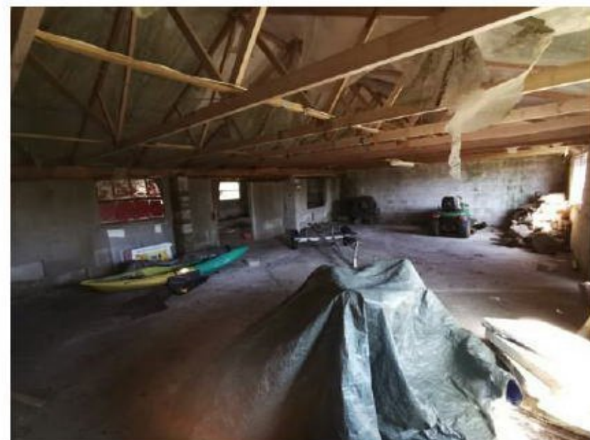
Photo 6. Showing the interior of building 2
