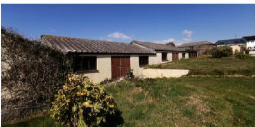
Photo 3. Looking up the eastern side of the building
