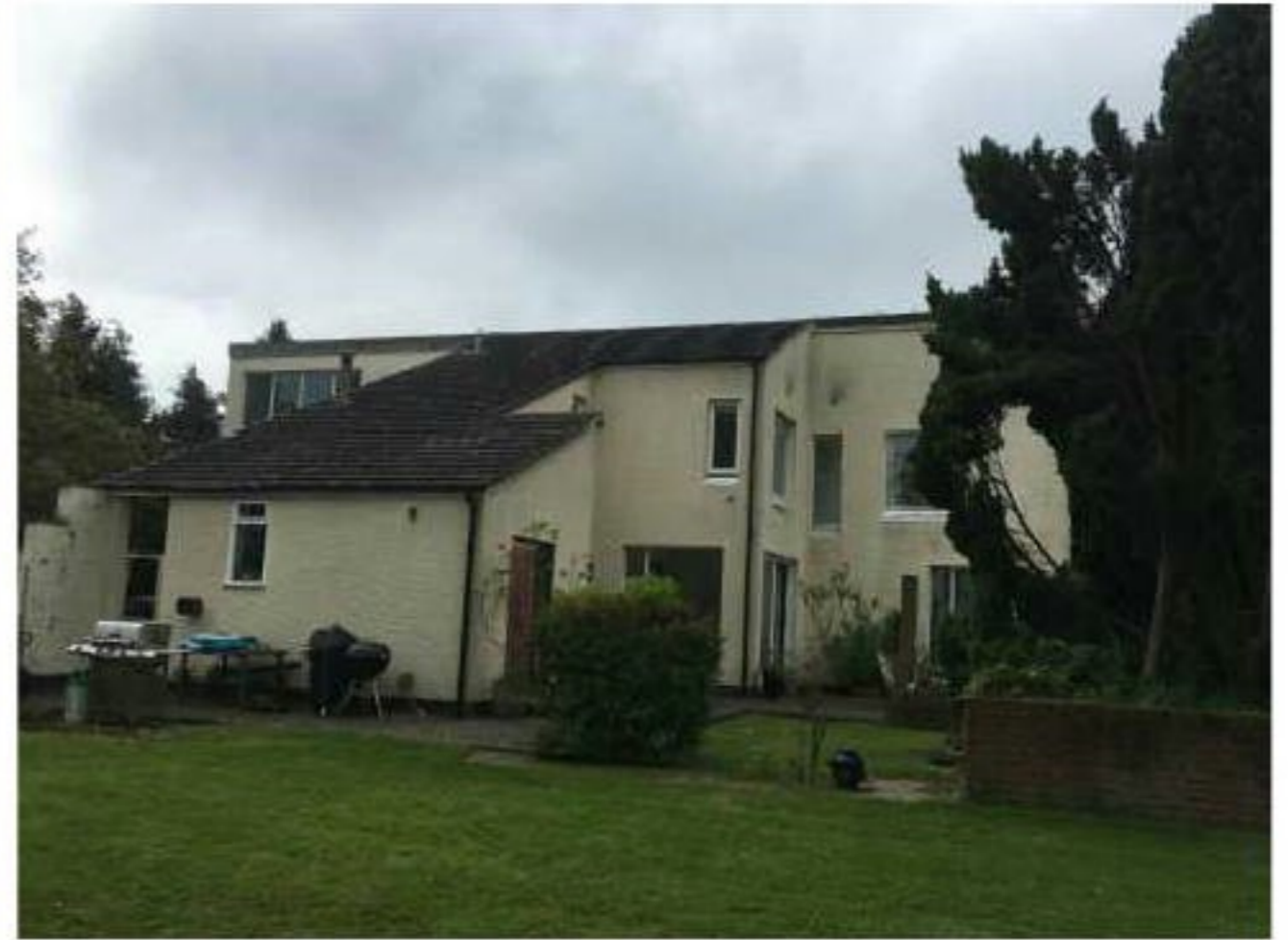
PHOTO: existing house north elevation
