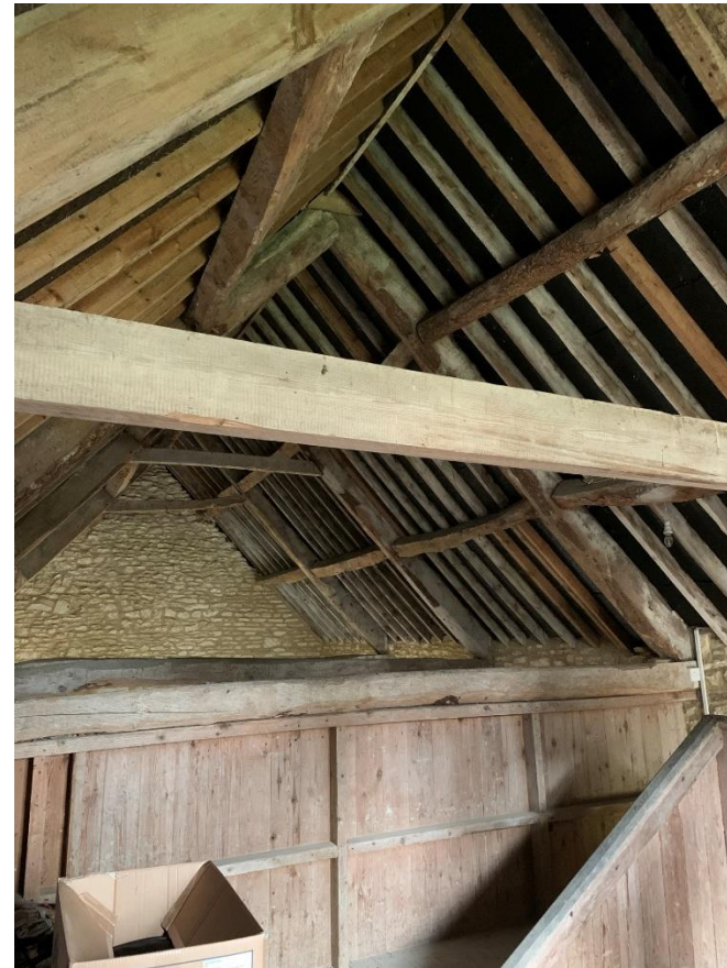
Mezzanine with altered truss in foreground
