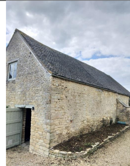
Photograph 2 – north-east aspect of B1
