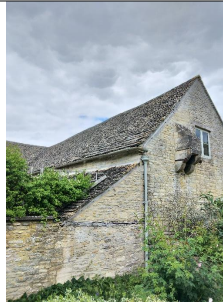
Photograph 5 – south-eastern aspect of B1.
