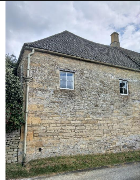
Photograph 4 – west facing gable end of B1.
