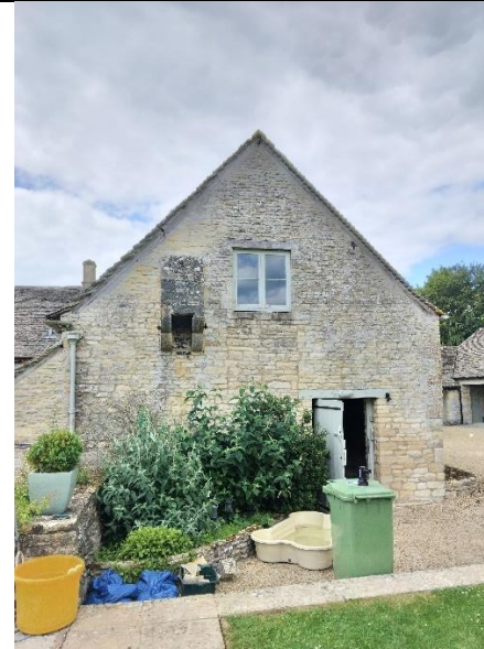
Photograph 3 – East facing gable end of B1.
