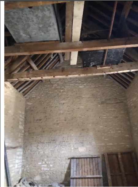
Photograph 6 – Internal view of the room within the west side of the
