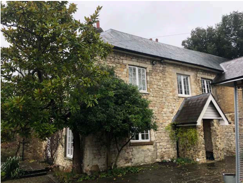
Fig 11- Corner view of rear and side elevation. Note: Magnolia tree, level changes in terrace
