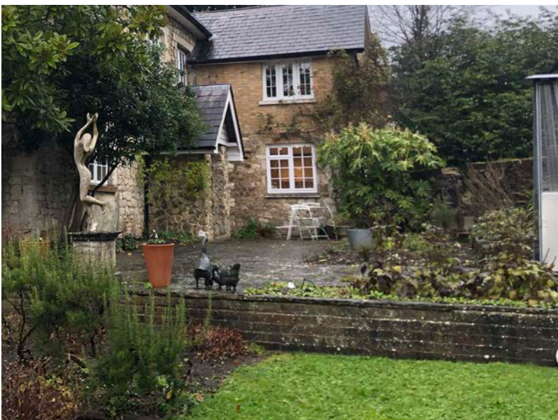
Fig 12- Corner view of rear and side elevation. Note: level changes in terrace
