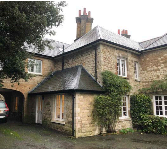
Fig 7- Single storey extension built in 2001 to accomodate utility room
