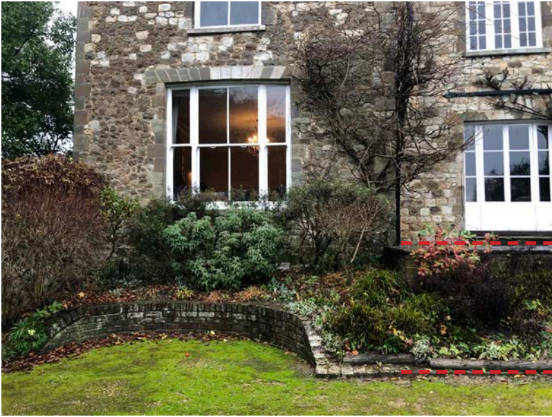
Fig 10- Rear Elevation. Note: Height difference between patio and garden
