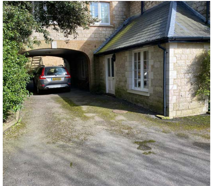
Fig 8- Single storey extension built in 2001 to accomodate utility room
