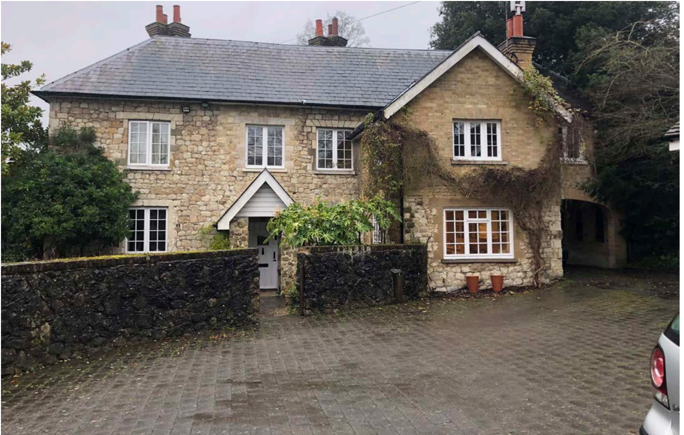
Fig 3- Side Elevation view, entrance vestibule. Archway to the right leads to the original front entrance. Note: window above the entrance appears to have relocated over the years. The proposal is to reinstate it to sit centred on the ground floor corridor.
