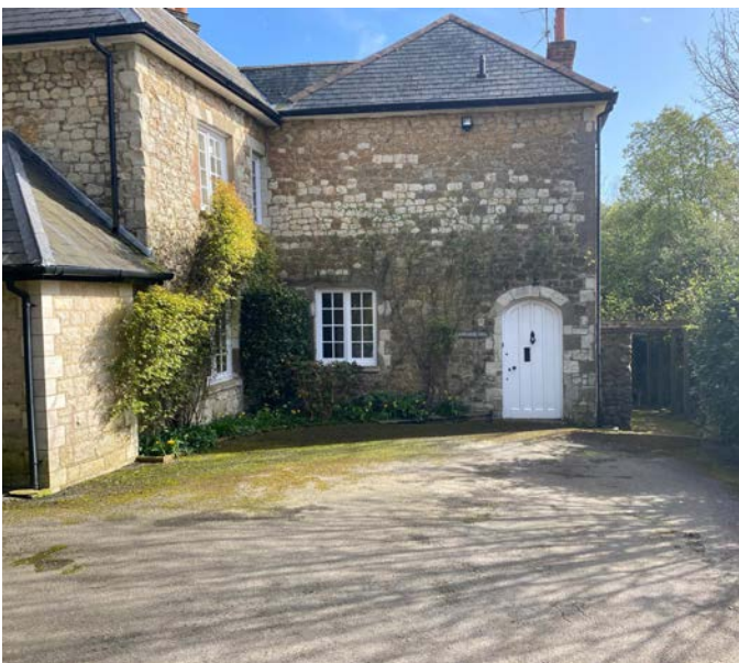
Fig 9 - Front elevation. Original front door.
