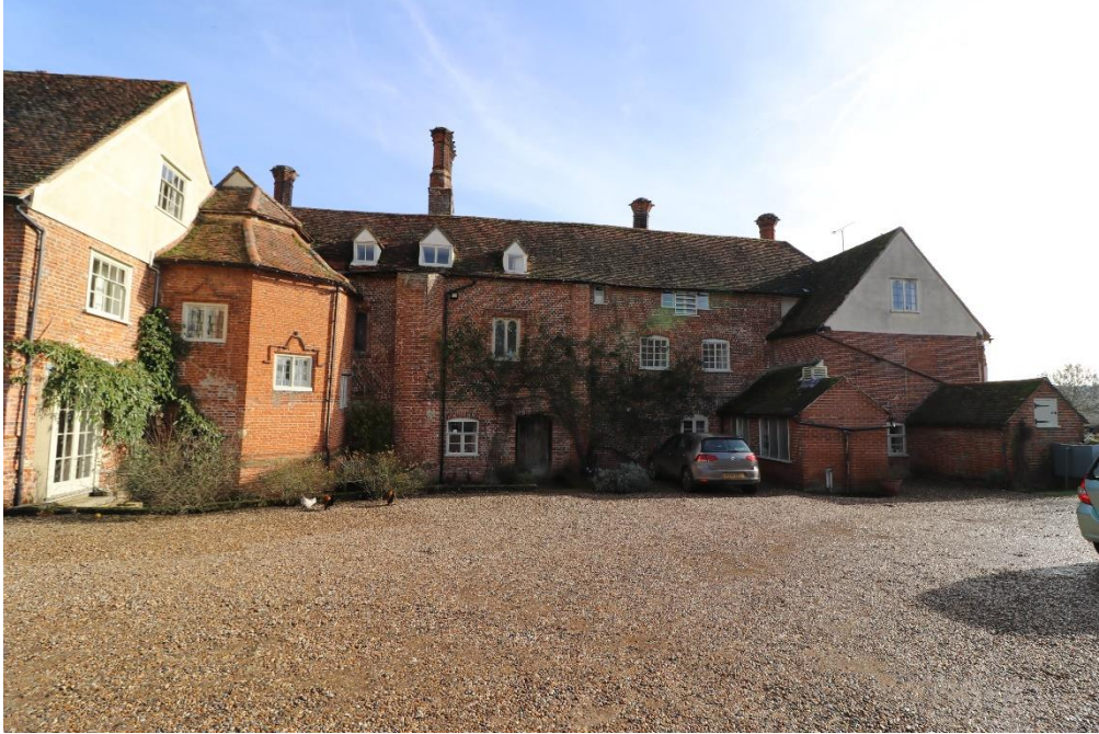
Photo 2. Shelley Hall west elevation.
