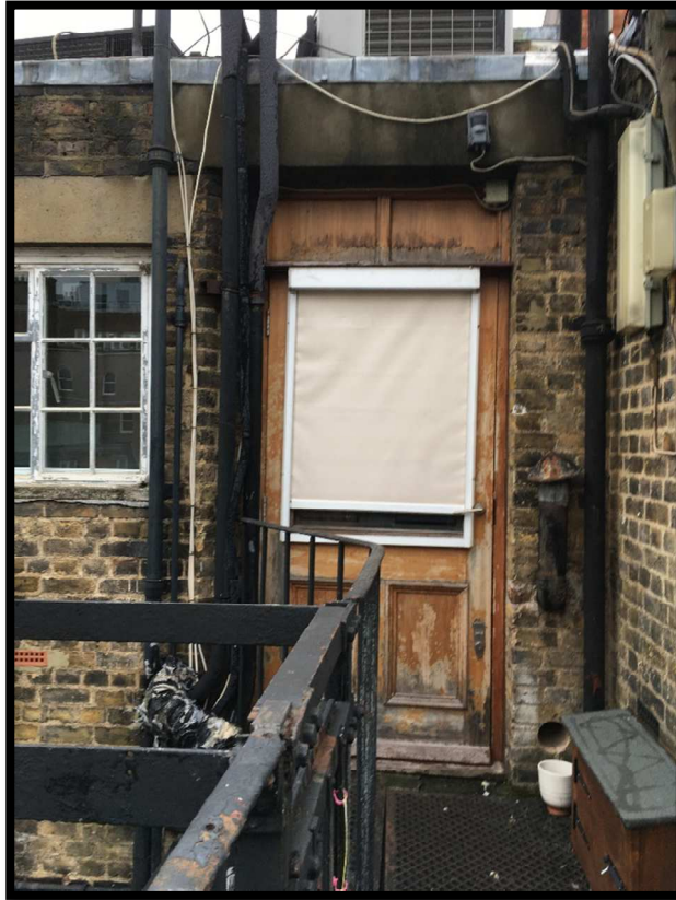
Disused top floor egress door to be replaced
