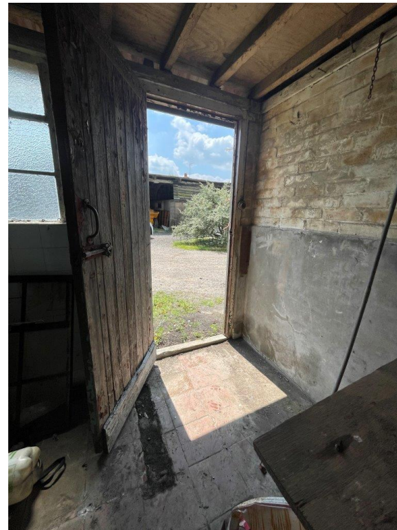
Access into mens WC
