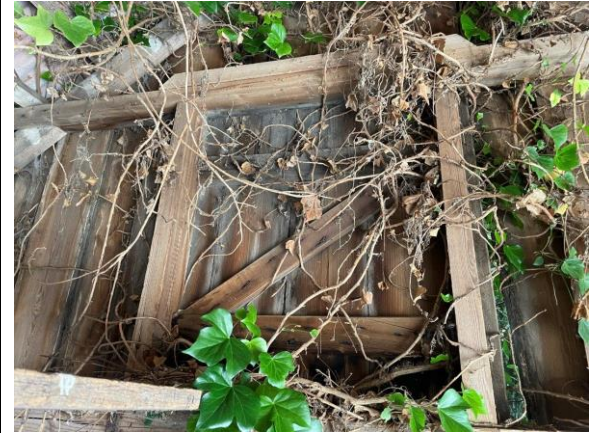
Timber hatch in top of east gable
