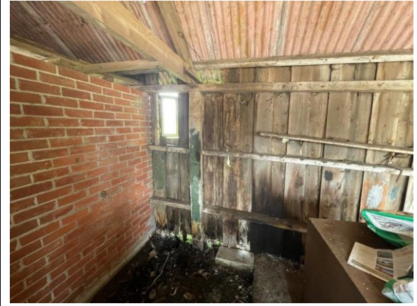
Open store internal elevation facing north. Next to mens WC area
