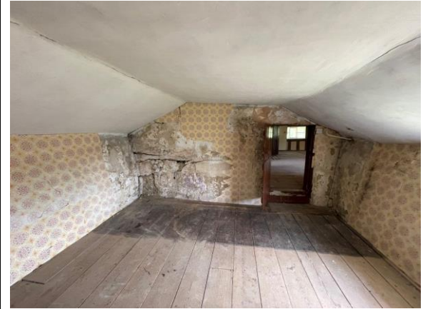
Internal elevation facing east
