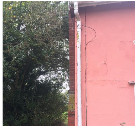
Severe linear crack / movement to corner of south elevation and west elevation. Running from ground to eaves.
