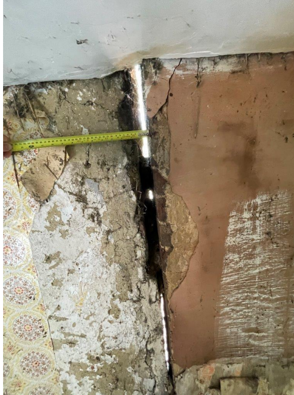
Cracking between west and south walls, evidence of walls splaying out by latter infill timber strips to perimeter of room. Bearing of floor joists in walls and condition questionable.
