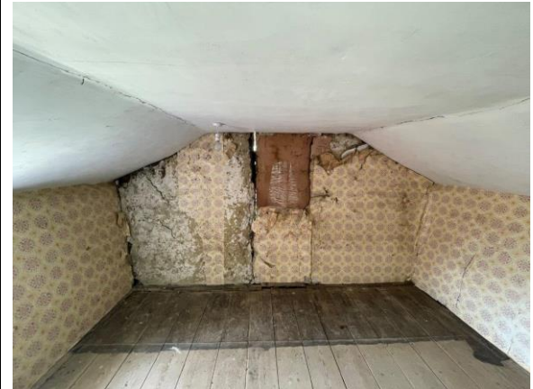
First floor facing west, movement between clay lump and masonry chimney evident, daylight clearly visible.
