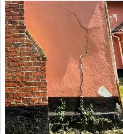
Severe crazing to west elevation south and north of chimney breast
