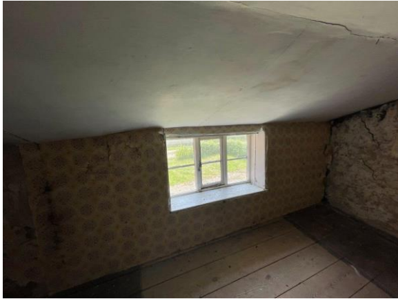
First floor window to south
