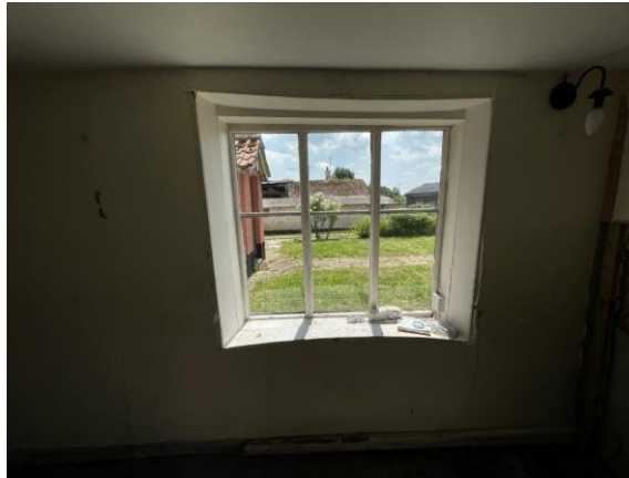
Ground floor window to south, saturated plinth shows swelling and movement evident by warping to cill and head of window
