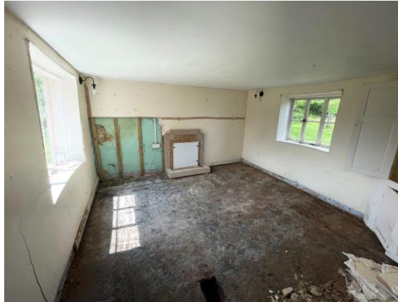
Ground floor window to south, saturated plinth shows swelling and movement evident by warping to cill and head of window
