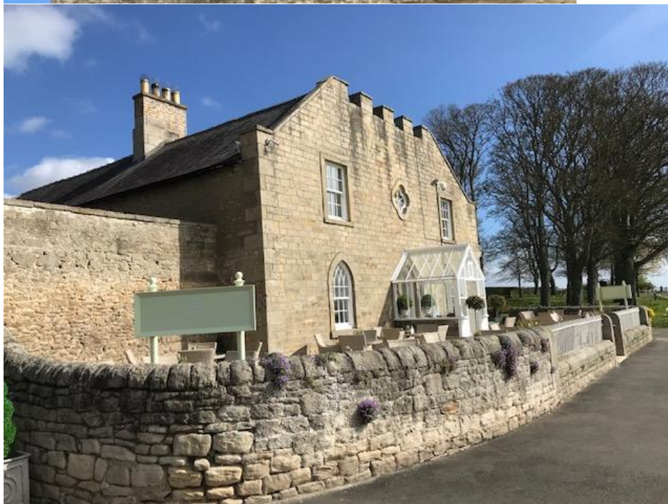
Figure 9: Camera 2: CCTV camera to front of Unit 3 (close up above)
