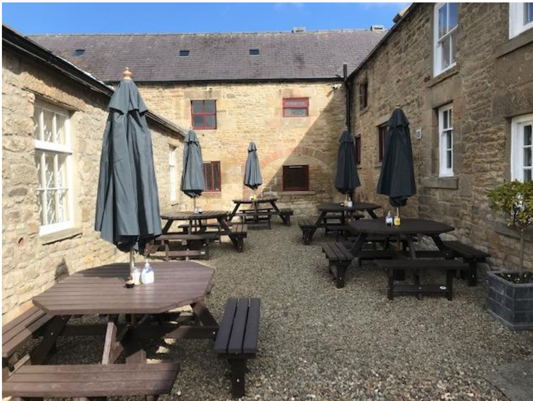
Figure 12: Hemmel arch in Unit 7 proposed for opening in a style similar to Unit 10 above
