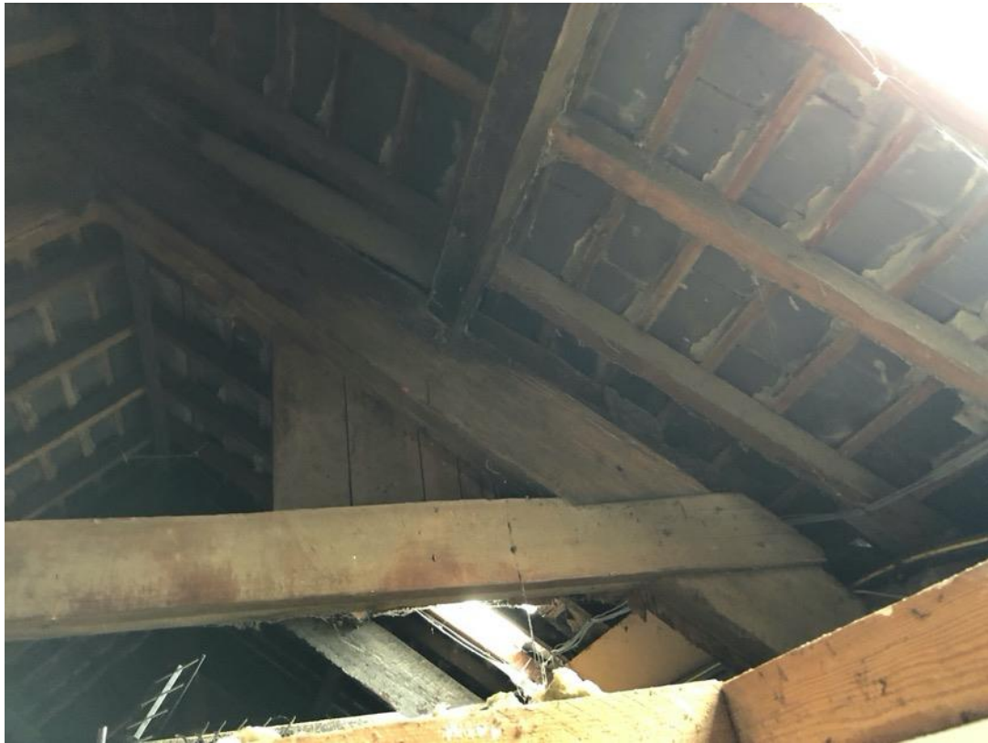
Figure 15: Rafters in loft space (Unit 7) to be revealed and restored
