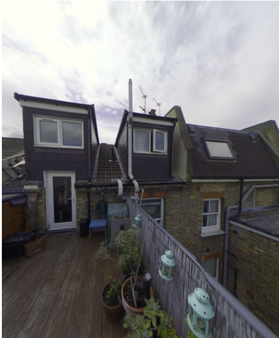
Figure 3, rear elevation view
