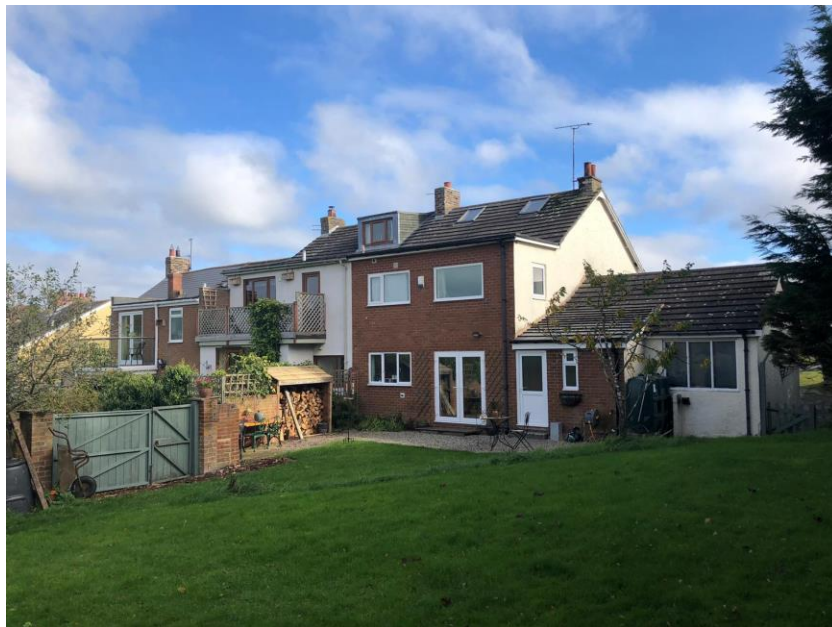
Existing access gate and hardstanding to the rear of the property
