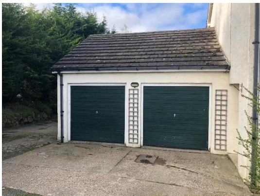
Existing double garage
