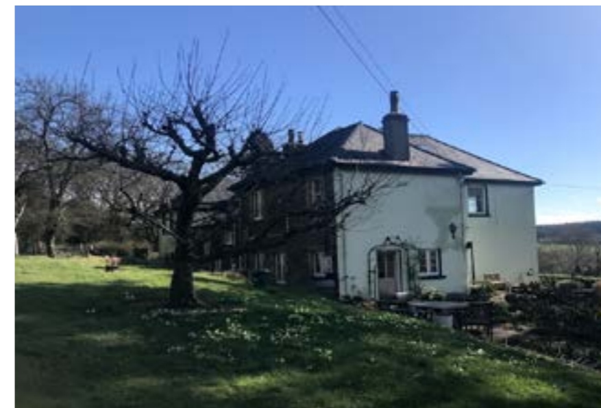
East elevation of Hunter's Lodge
