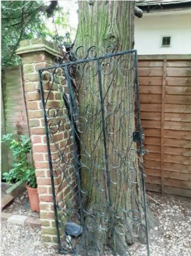
Figure 1 image of actual damage caused by T005 trunk
