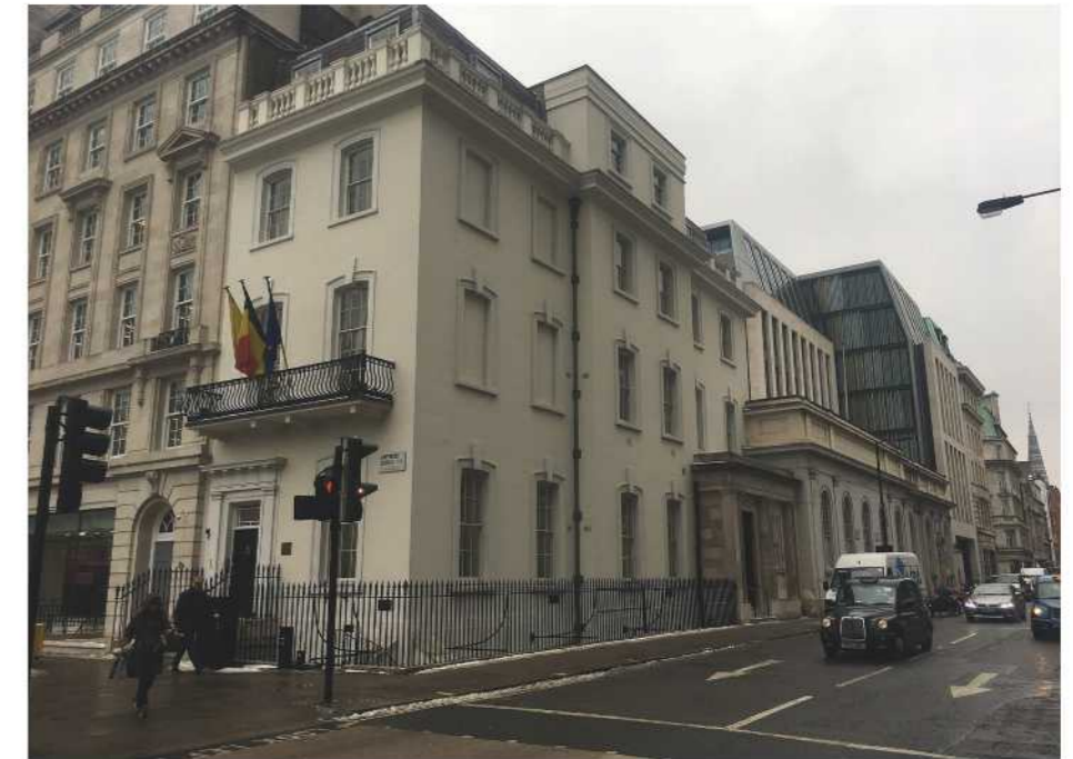
Figure 4.1 Site looking east along Margaret Street
