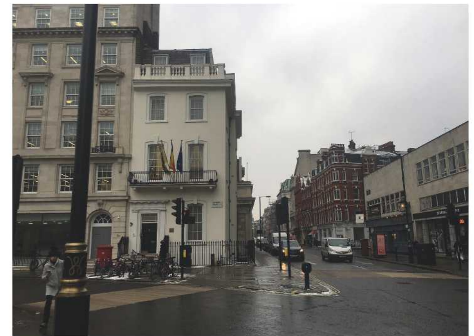
Figure 4.2 Site looking east from Cavendish Square
