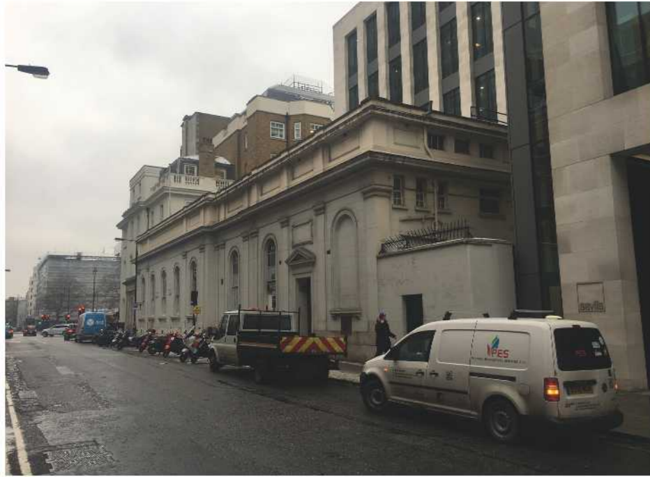
Figure 4.4 Site looking west along Margaret Street
