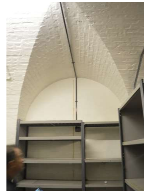
F: Vaulted piers and infill
