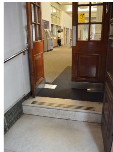
E: Entrance steps
