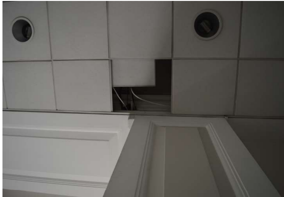
A: False ceiling with cornicing hidden (looking up)
