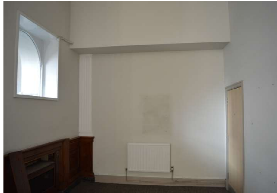
B: End wall infilled to separate properties
