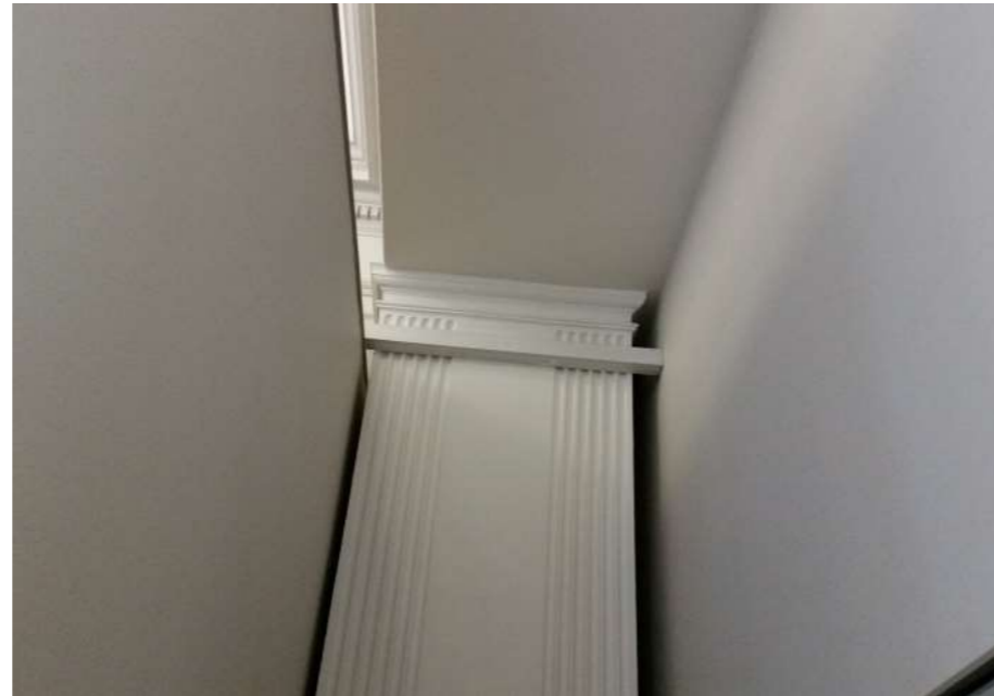
B: Pilaster sandwiched between stud walls
