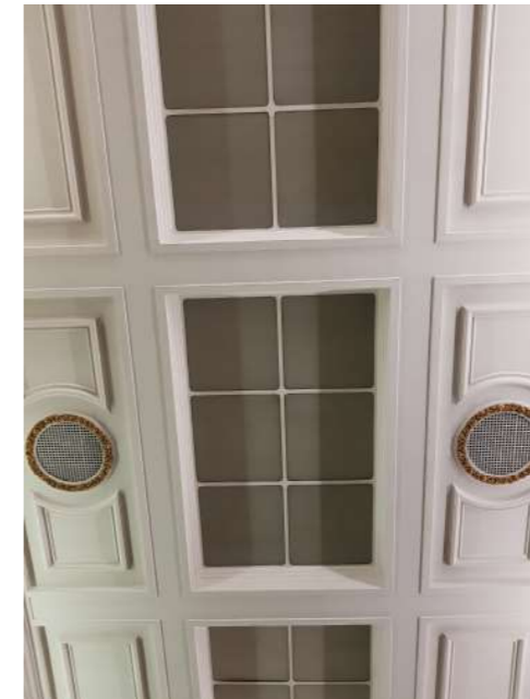
C: Ceiling with lighting (looking up)
