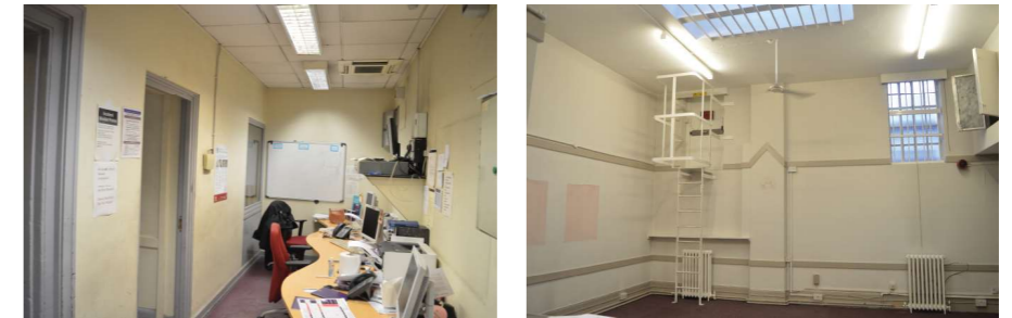
C The east wing has been historically altered to serve the changing functions for the bank. Modern alterations, particularly at first floor level and to the service areas detract from the historic character and confuse legibility of this space.
