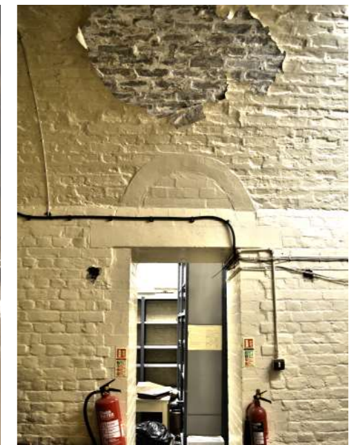
G: Altered entrances to brick vaults
