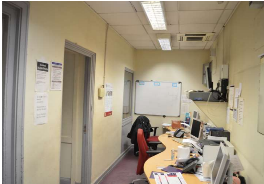
A: Offices area with stud walls and false ceilings
