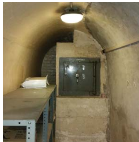
Photograph showing vaulted area.
