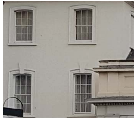
Photograph of existing windows
