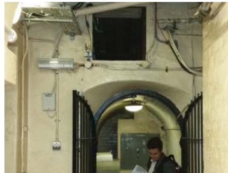
Mechanical void above vault
