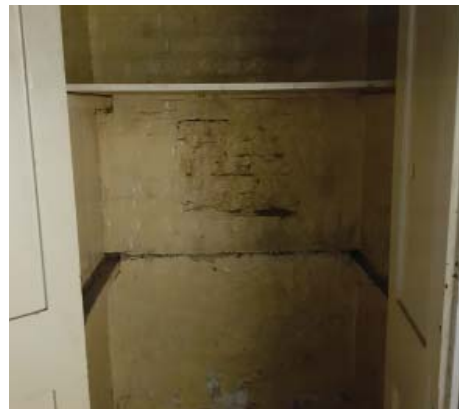
Photograph showing location of existing opening to be reinstated
