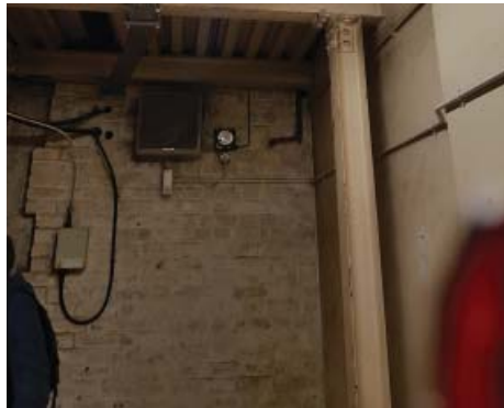
Photograph of brick infill to lightwell
