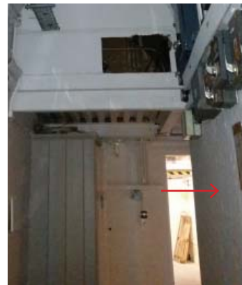
Photograph showing stairwell wall with services to the right.
