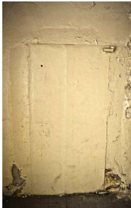
Photograph showing recessed infill of original opening
