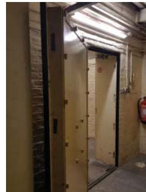
Photograph showing existing opening
