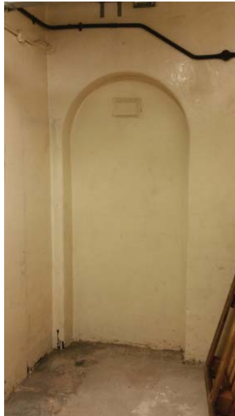
Photograph showing recessed infill of original opening
