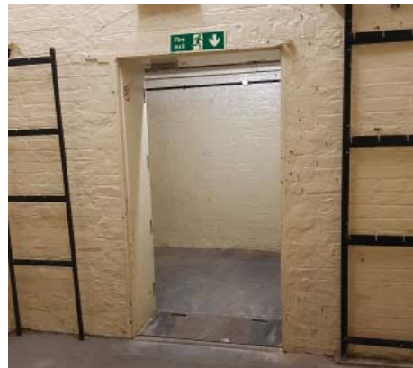
Photograph showing existing proportions of opening to be formed.
