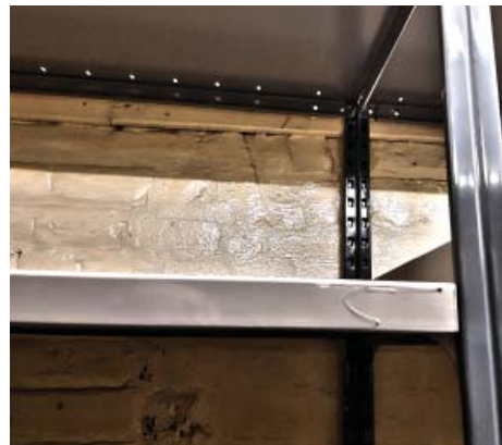
Photograph showing new brick joining to existing vault
