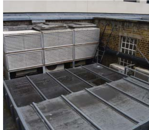
Photograph showing redundant services units and concealed skylight
