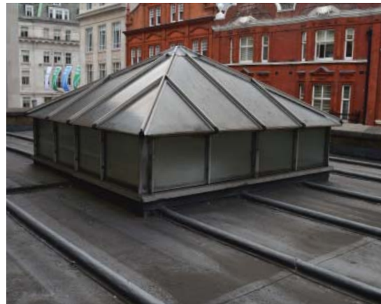
Photograph showing aluminium skylight
