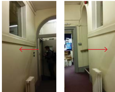
Photographs showing wall to stairwell
