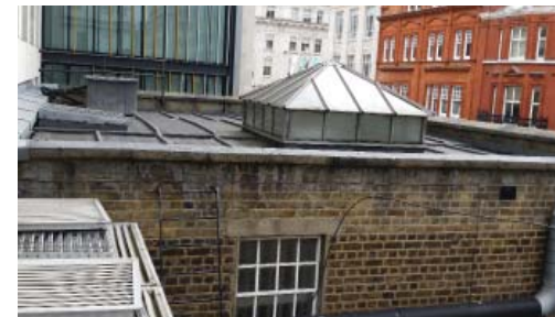
Photograph showing roof area
