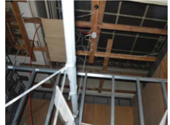
Photograph showing skylight concealed within service void in false ceiling (looking up)
