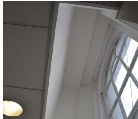
Photograph showing arch window truncated by false ceiling
