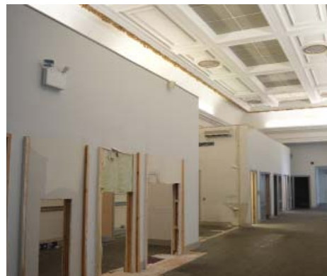
Photograph showing modern stud partition walls to be removed
