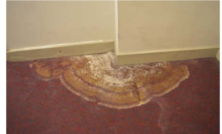
Photograph showing mould spread
