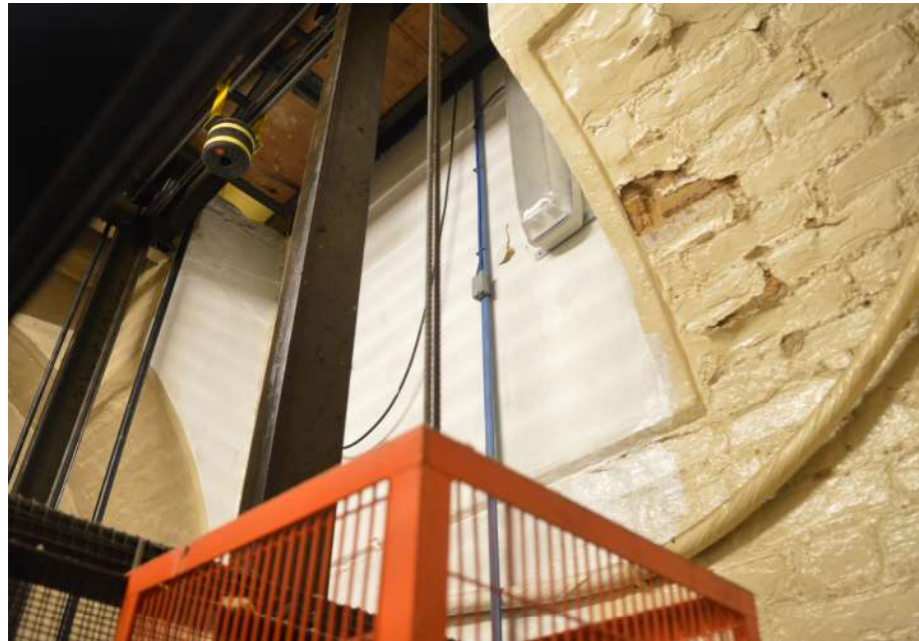
A: Lift shaft cutting away vault opening
