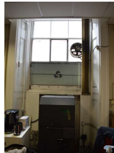
E: False ceiling through window
