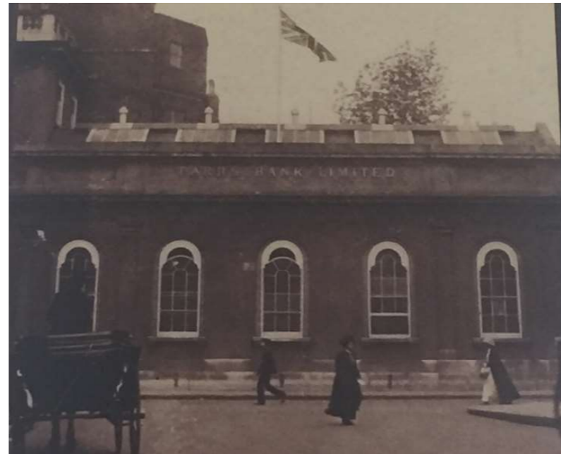
Circa 1900: Parr's Bank with sash covered arched windows, a raised ridgeline to the pitched roof with skylights and less frieze detail
