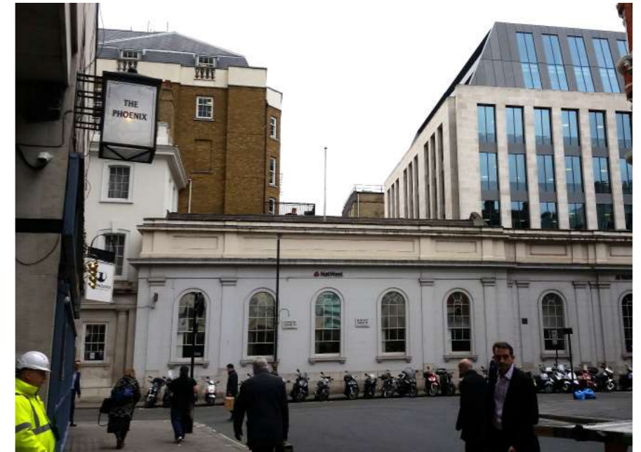
2016: Existing condition as Natwest Bank with arched windows, pitched roof with skylights and chimney stack and a noticeable difference in stonework
