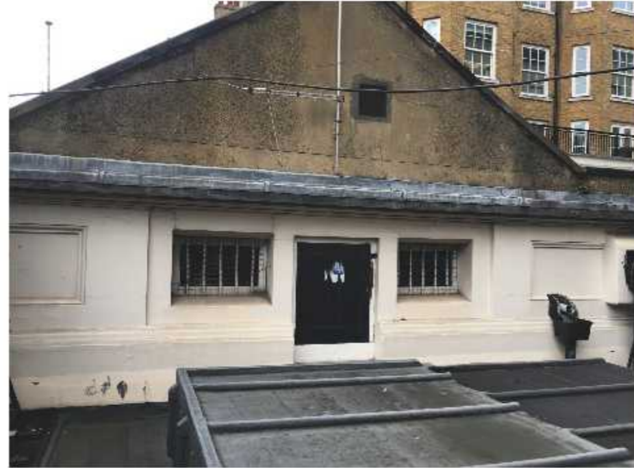
Figure 4.11 External east facing gable to Banking Hall roof
