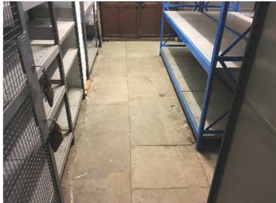
Figure 4.16 Flag stones to basement
