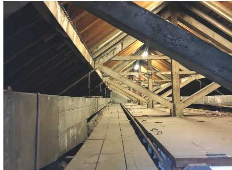
Figure 4.12 Roof structure above Banking Hall
