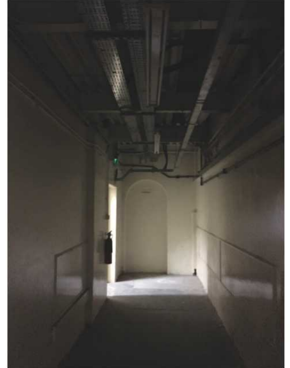
Figure 4.17 Hallway in basement
