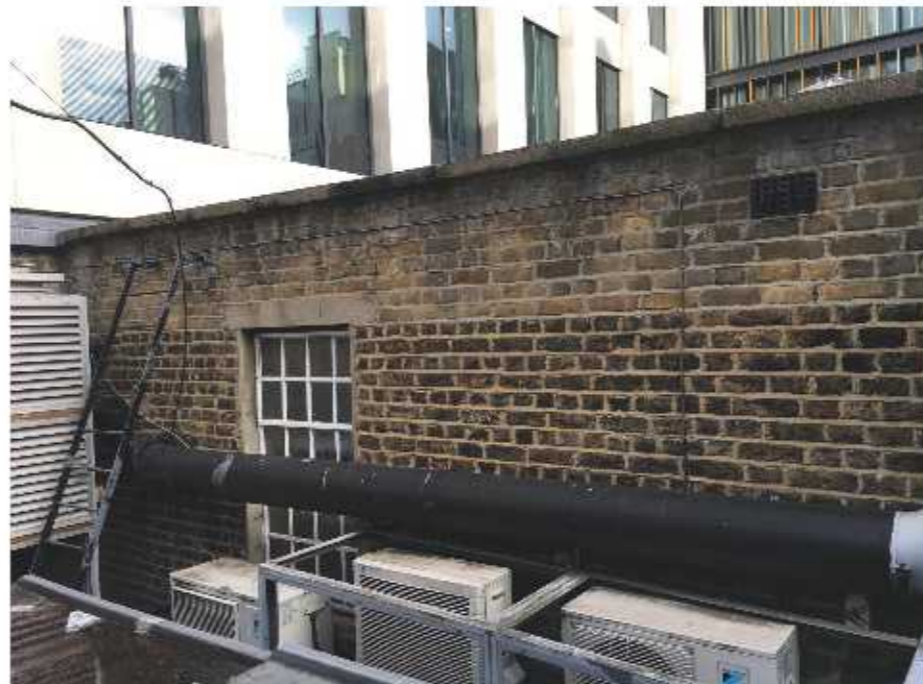
Figure 4.23 West facing wall to first floor
