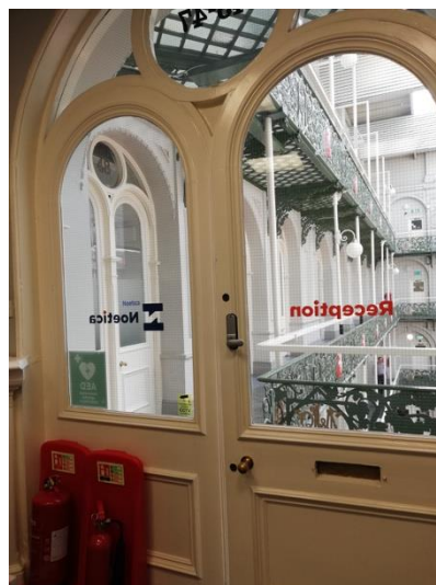
Image 49: Typical door and window opening onto atrium which maximises light from roof into offices.
