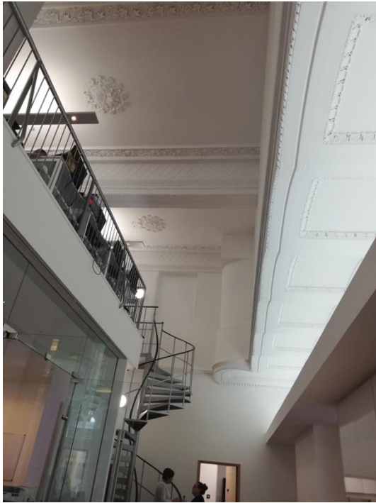
Image 35: Decorative ceilings and cornice in former subscription rooms
