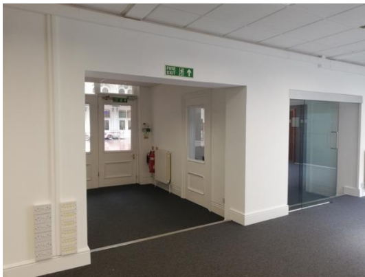
Image 37: Transition from trading floor through original offices into modern Atrium Suite
