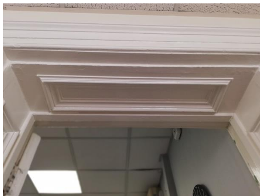
Image 46: Illustrates retention of original detailing despite insertion of suspended ceilings
