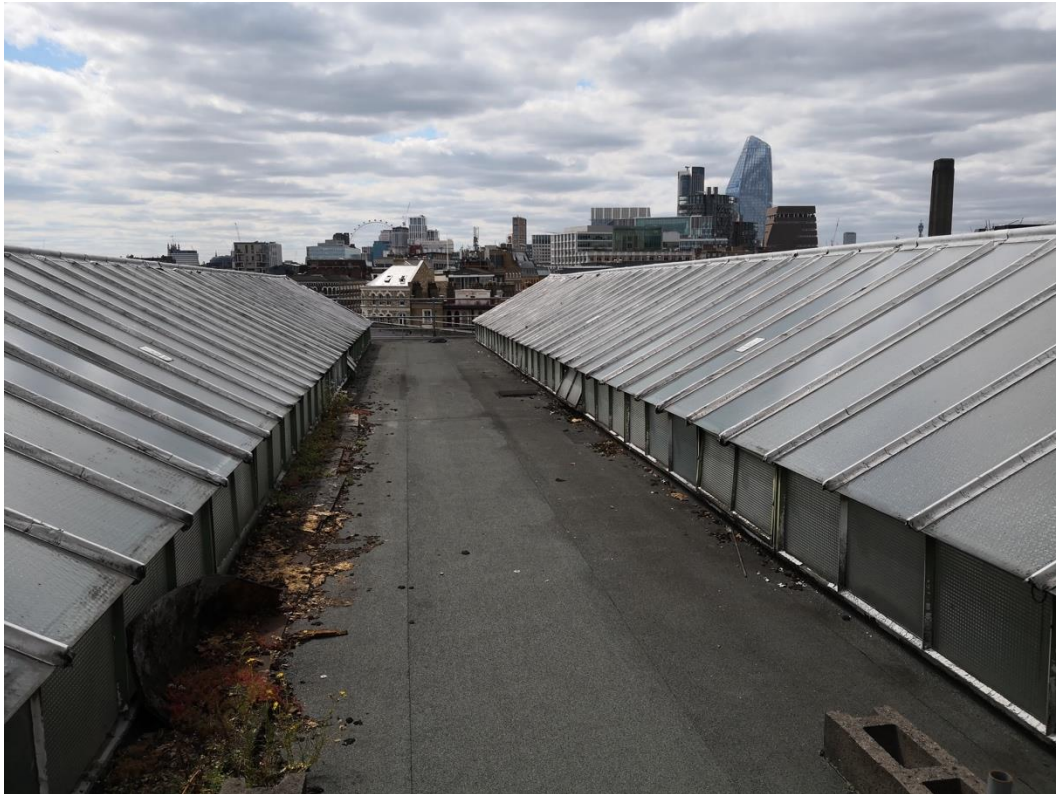
Image 59: Atrium Roof (1970s)
