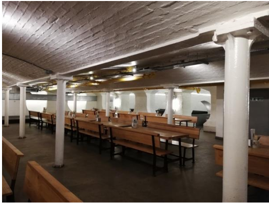
Images 18 & 19 (above) Basement Cellar beneath trading floor with cast iron supports. The cells around the edge lie beneath the trading floor offices.
