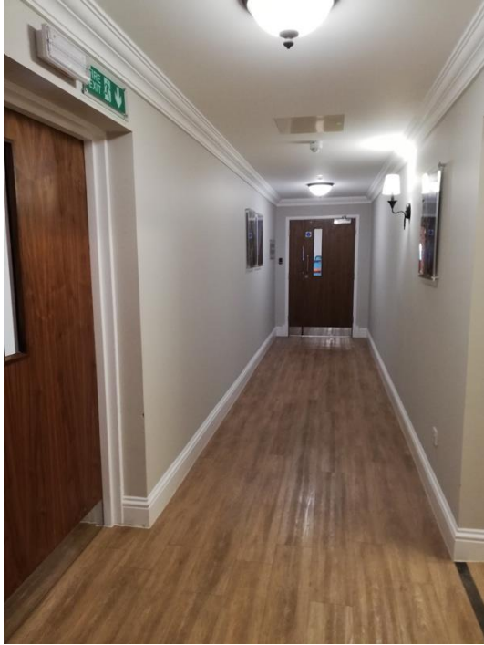
Image 32: Lower Ground floor corridor: modern fit out obscures original structure
