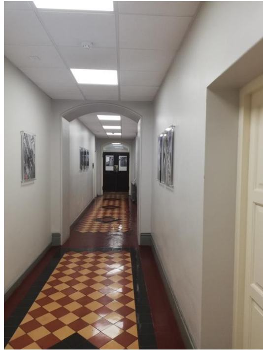
Image 36: Corridor to West Wing with original shape, form and floor but modern ceilings, doors and decoration
