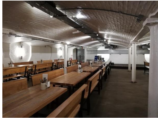
Images 18 & 19 (above) Basement Cellar beneath trading floor with cast iron supports. The cells around the edge lie beneath the trading floor offices.
