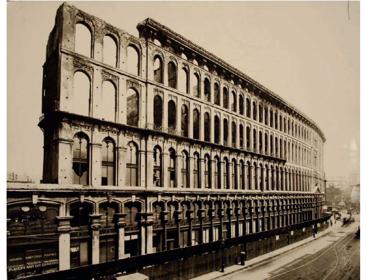
Hop Exchange post fire in 1920 showing burnt out top two storeys
