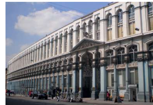
Image 4: Principal façade, Southwark Street
