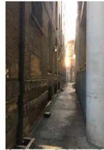
View 4 - narrow alley between rail viaduct and building
