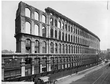
Photograph post fire
