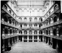
Atrium internal photograph
