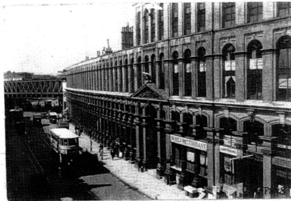
Figure A5 – 1931 – Elevation reduced to two arch tiers on west side of structure
