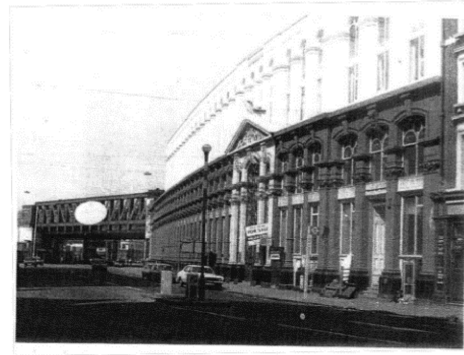
Figure A7 – no date – Elevation reduced to two arch tiers across full front elevation
