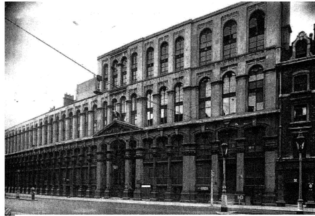
Figure A6 – no date – Elevation reduced to three arch tiers on east side of structure
