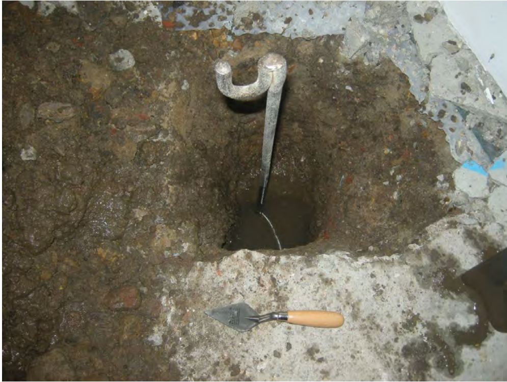
Photo 9 TP 8, against a footing in a room in the lower basement, looking south-westwards
