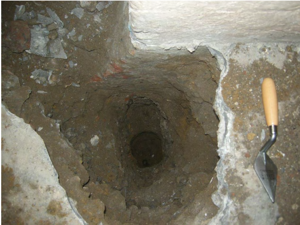
Photo 11 TP 10, in the coal cellar passageway, against a footing, looking northwards
