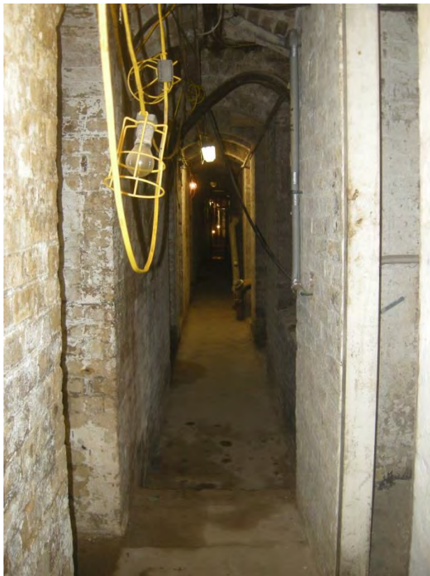
Photo 14 The coal cellar passageway, looking westwards from the stairwell towards TP 1
