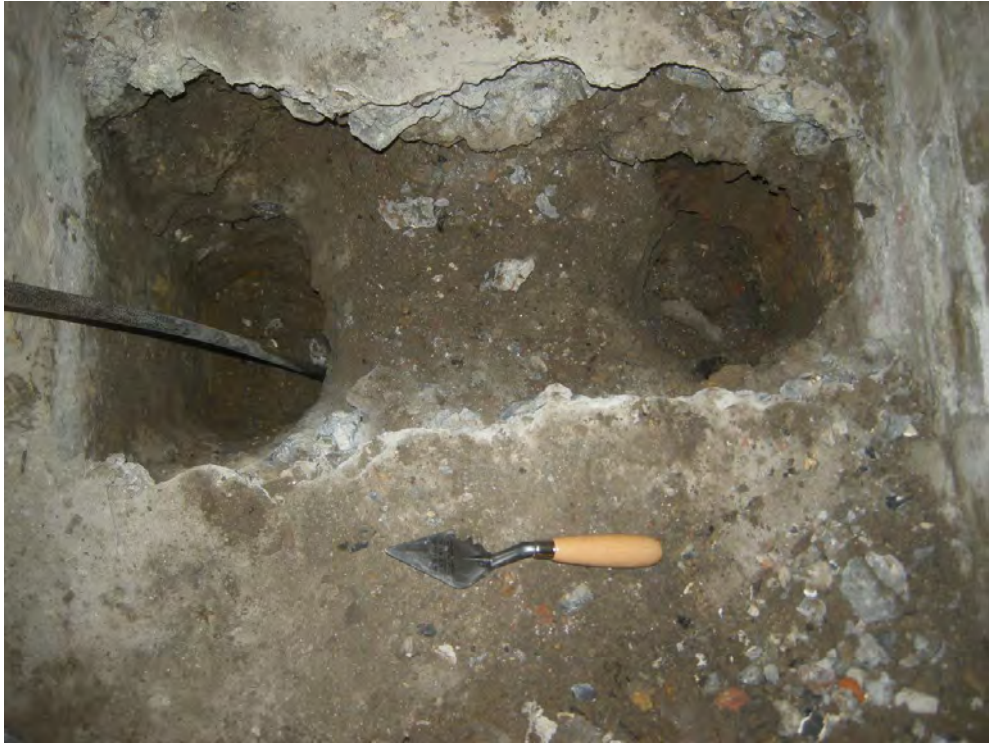
Photo 1 TP 1, in the coal cellar passageway, between the footings, looking eastwards
