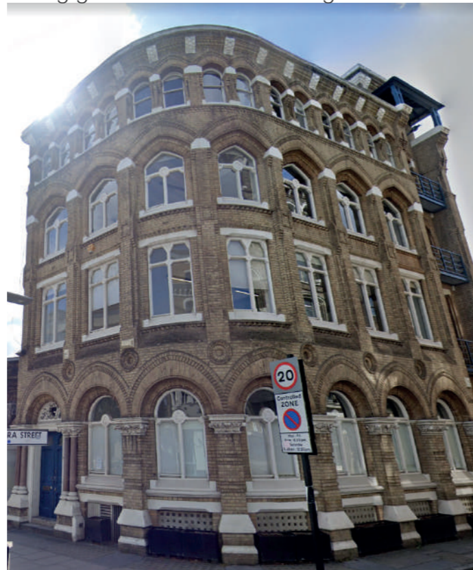
49 Southwark Street Yellow stock, parapet roof, arched windows, strong verticality and horizontal elements
