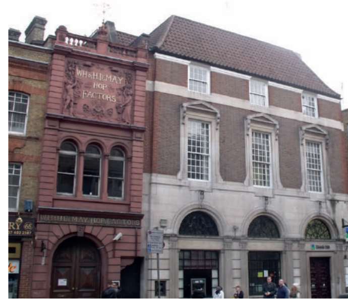
67&69 Borough High Street Arched windows, decorative elements and parapets
