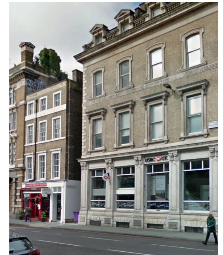
28 Borough High Street, Yellow stock, parapet roof with loft floor and a strong grid
