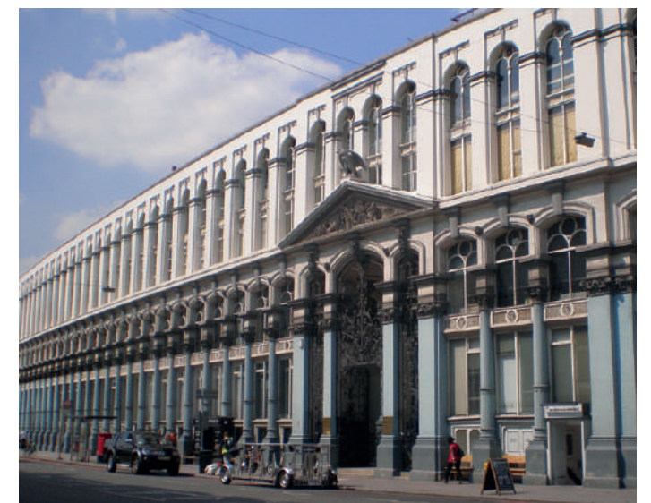
View 5 - Looking north-west towards the Hop Exchange building
