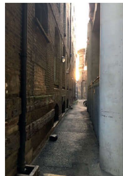
View 4 - narrow alley between rail line viaduct and building
