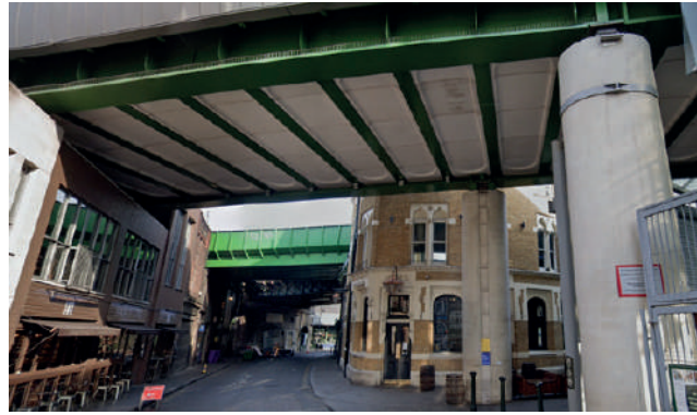
Bedale Street looking beneath railway bridge
