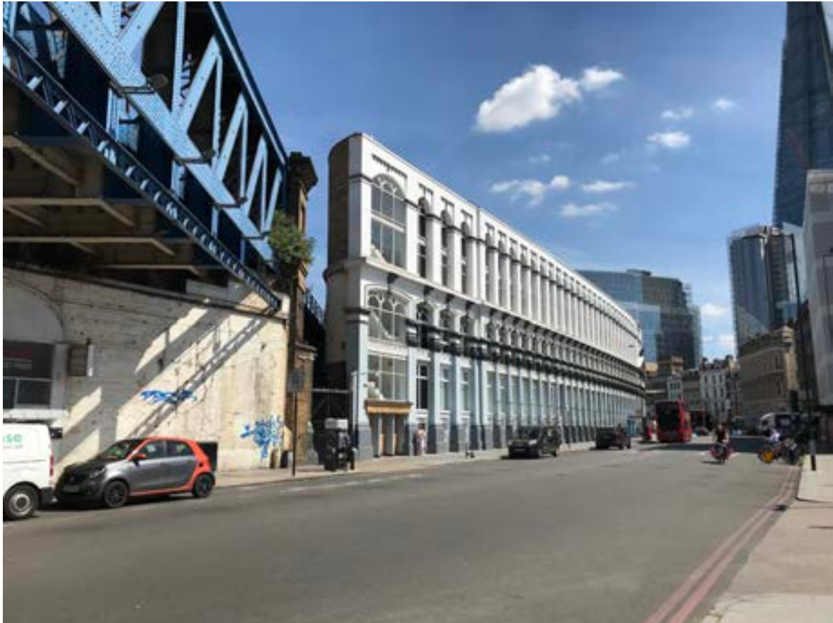
Plate 3: 2020 general Southwark Street Hop Exchange façade view eastwards
