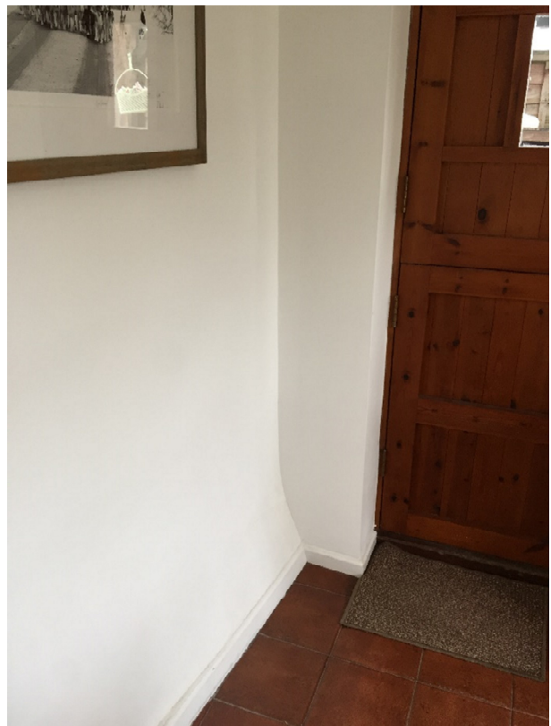
Image 08 – original wall junction noticeable by camber at bottom
