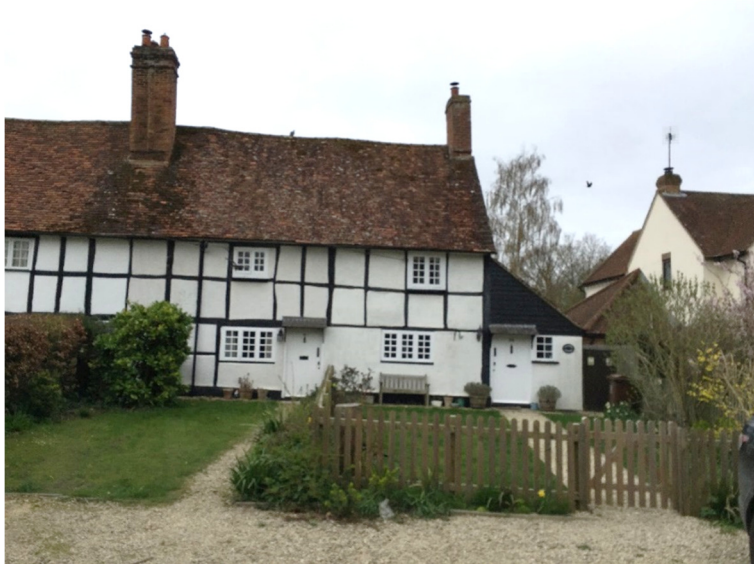
38 The Avenue (Front elevation, 38 The Avenue to the RHS/ end of terrace)
