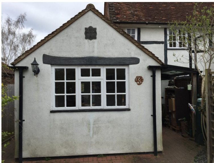
38 The Avenue west/rear elevation showing single storey side and rear extension and timber lean-to.
