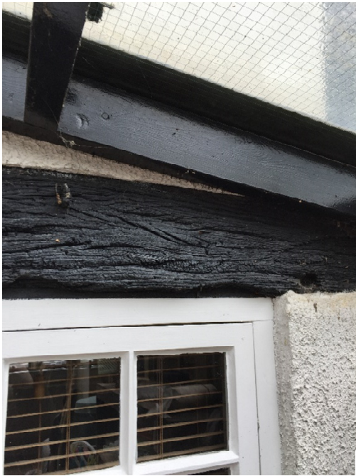
Image 06 – Lean-to fixed to original cottage
