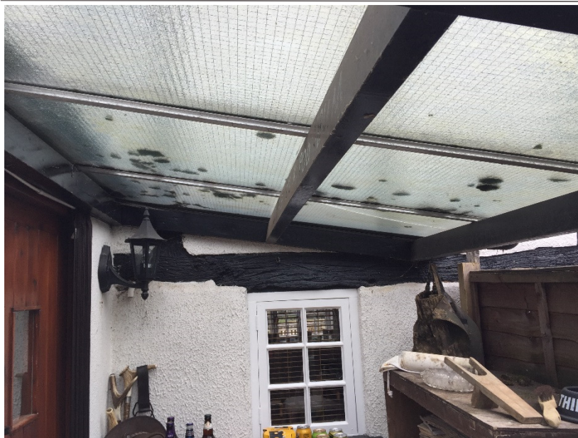
Rear elevation, lean-to abutting existing cottage and 1990's extension.
