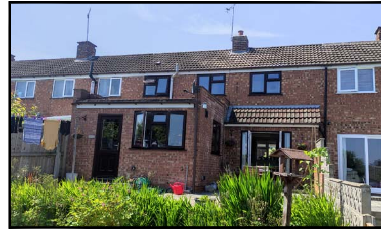
REAR ELEVATION PHOTOGRAPH
