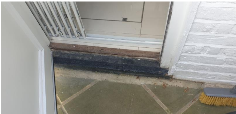
Evidence of Raised Floor
