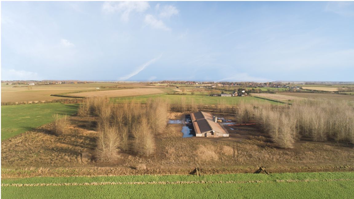
Picture 1 - Building before fire damage
