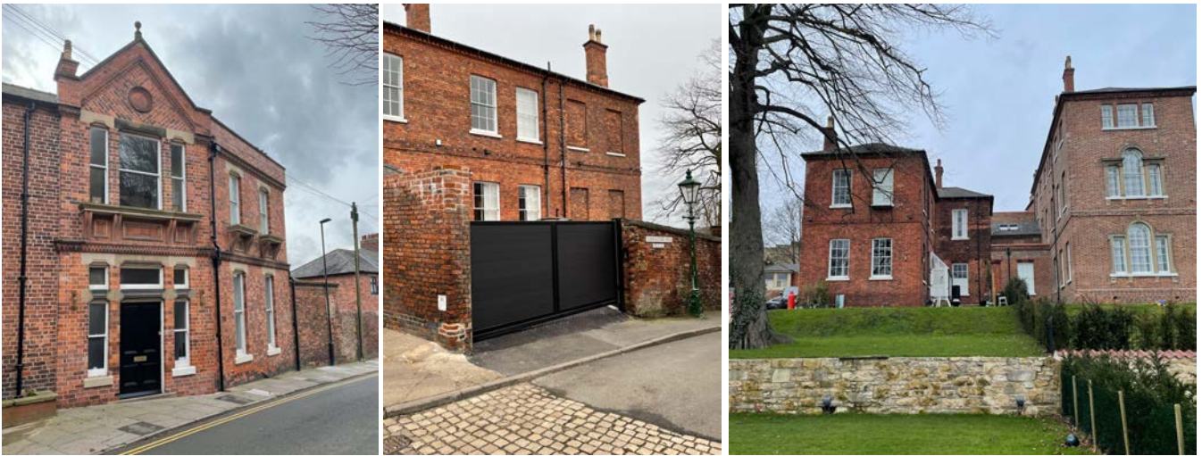
Fig 5: Front, side and rear views of the Wardens House
