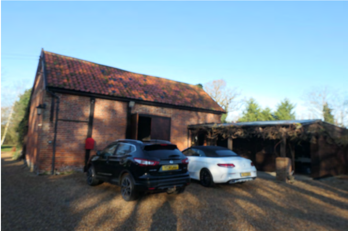
Photo 7 , south and east aspects of building one, looking north.
