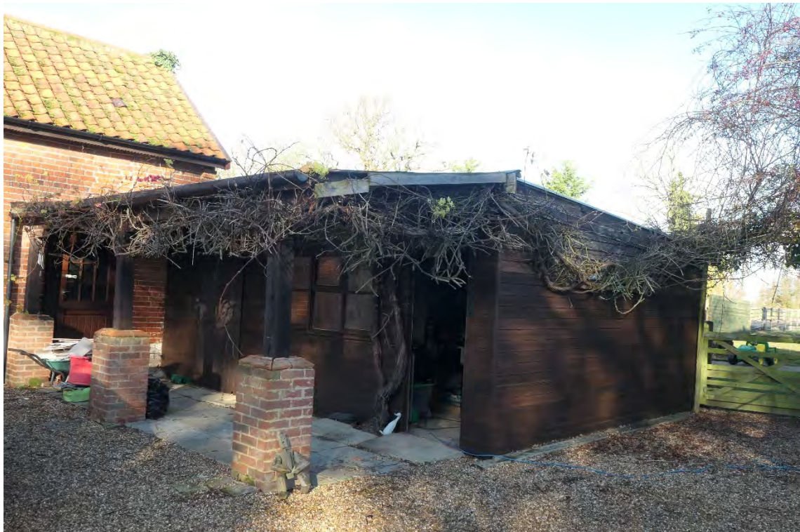
Photo 11 , south and east aspects of building three, looking north.
