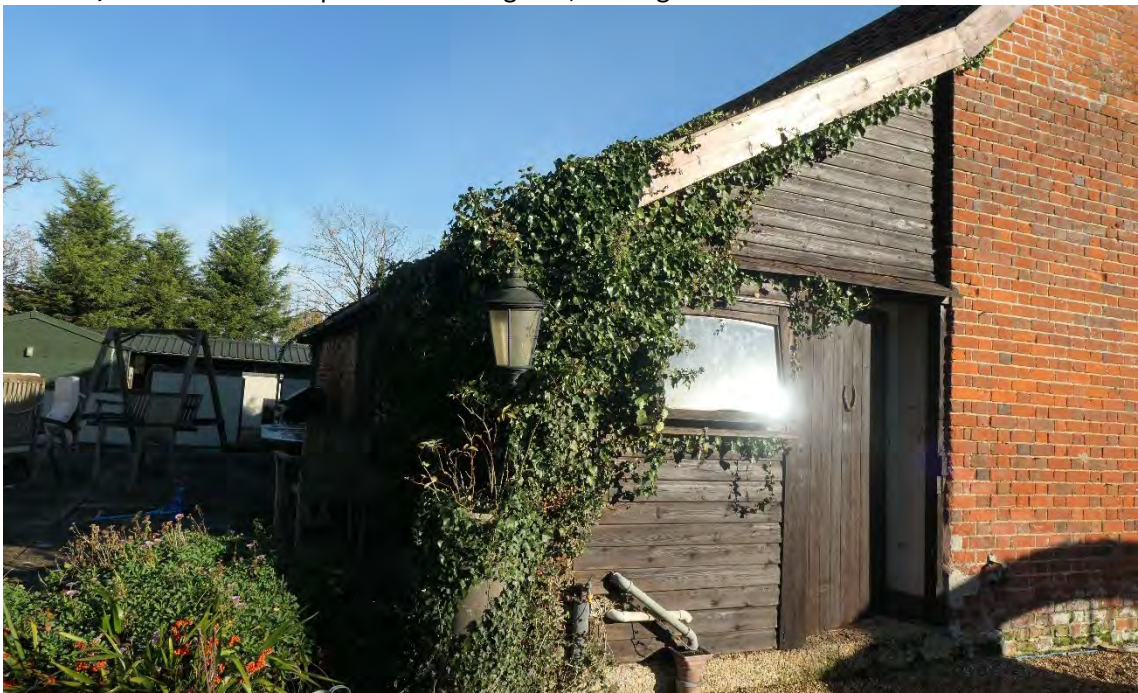
Photo 8 , section A of the barn.
