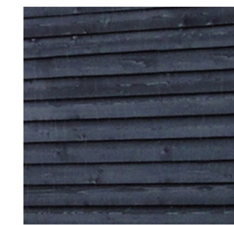
Black timber weatherboarding
