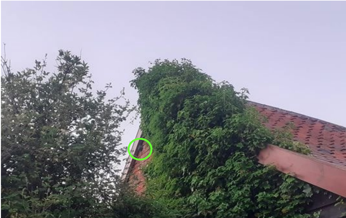
Photo 1 , brown long eared bat entered the building at 03:21 beneath a gap of the northeast gable timber fascia, indicated by green circle. 16 th June 2021.
