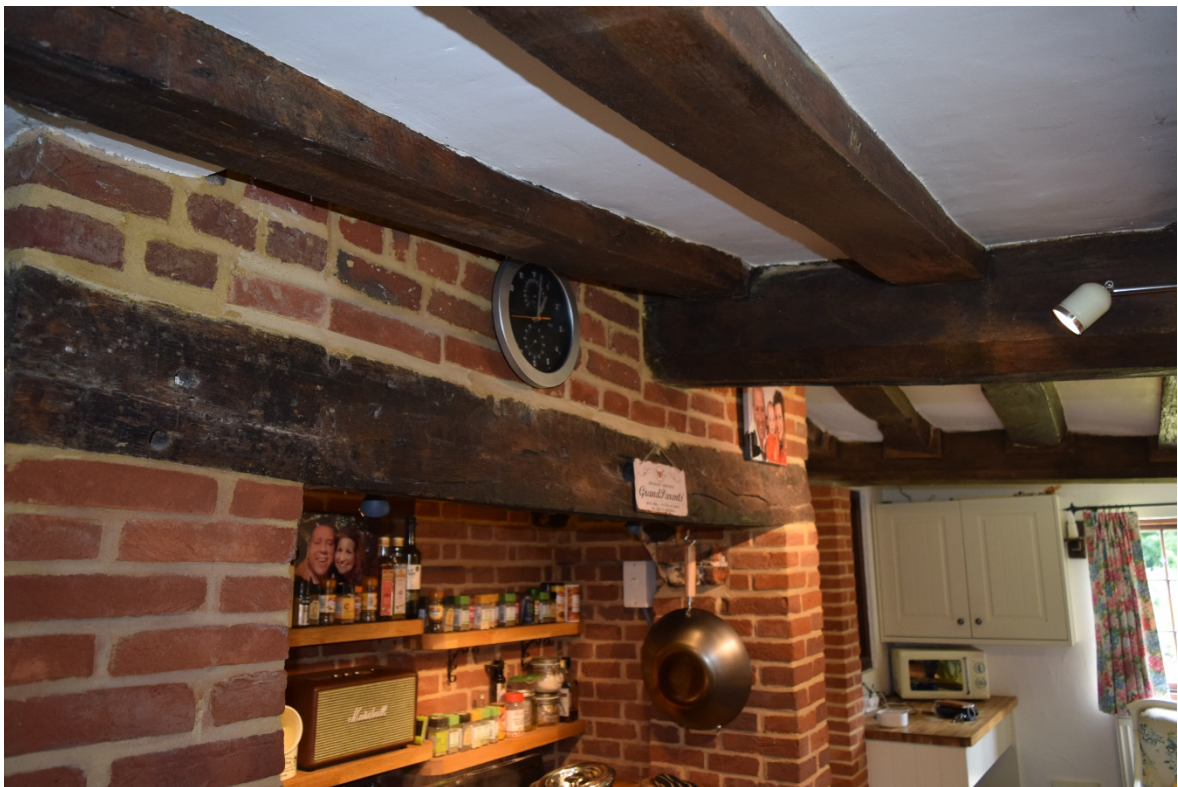
Figure 15: Floor structure over the kitchen.
