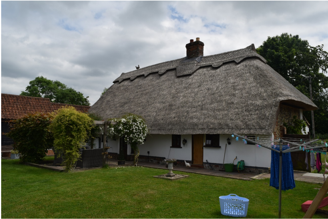
Figure 7: Rear (North) Elevation of Thatched Cottage.
