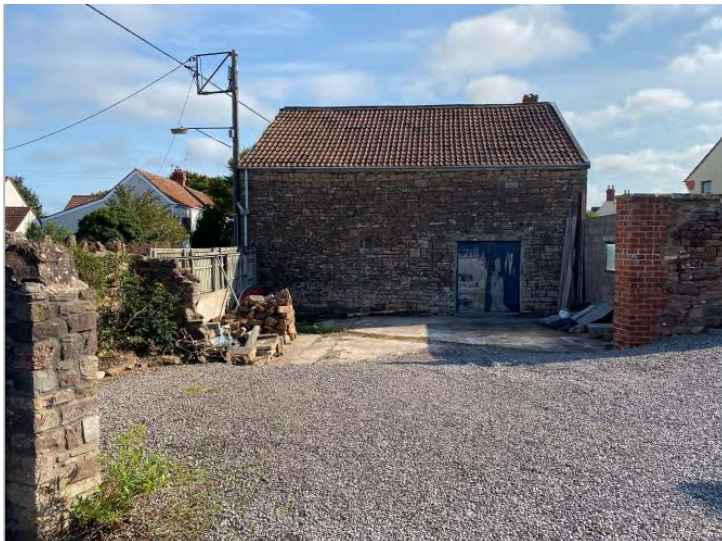
Front elevation of the existing stone outbuilding (to the left). Image Sourced: Collier Reading Architects.
