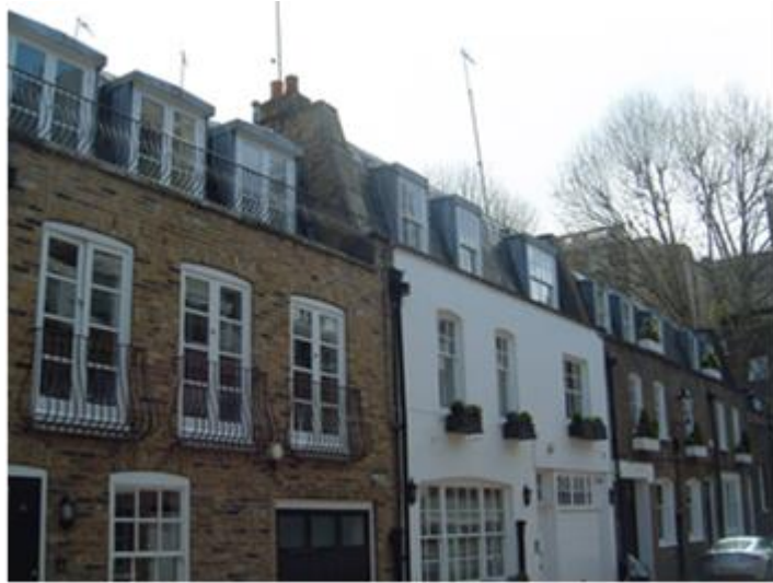
Figure 9 - No. 10 Albion Close with its mansard and front dormers is shown on the left of the photograph
