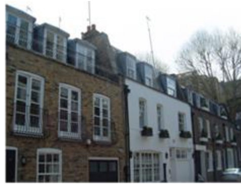
Figure 4 - View of No's 10, 11 and 12
