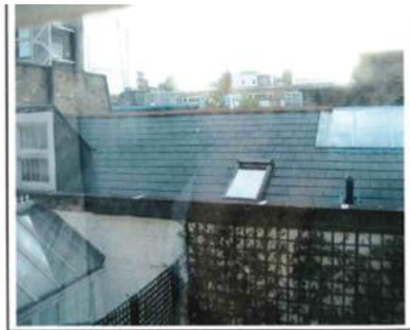
Figure 6 - View from 10 Albion Street looking west at the existing roof of the application site
