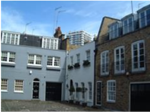
Figure 3 - View of No's 8, 9 and 10
